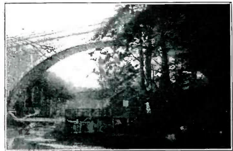
Cabin John Bridge, near Washington, forms part of the aqueduct system which supplies the city with water from the Potomac. It is 420 feet in length and the arch with a span of 220 feet, is the largest stone arch known.
