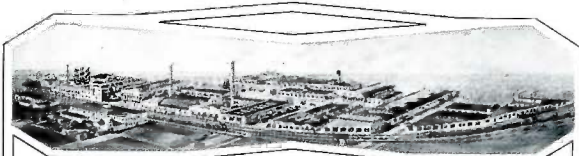
MAIN PLANT Decatur, Ill.
