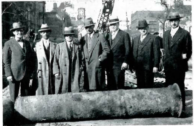
Section of a 24" cast iron main laid in 1854 and removed in 1932. This main, when removed, was in good condition and still serviceable.
