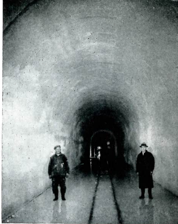
The new 16 foot tunnel 200 feet below lake level costing $13,500,000. It is now building and is known as Chicago Ave. Tunnel.
