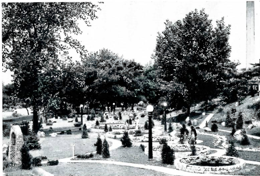
Beautiful grounds surrounding the Decatur Water Works Plant
