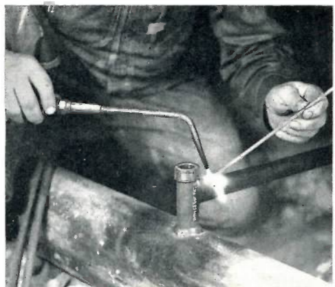
2. Main is cleaned, tee welded on, and service line is welded to outlet end of the tee.
