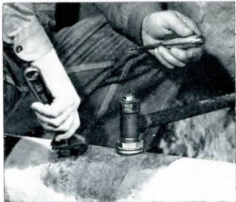
9. The service line is then connected to the tee. Machine-inserted No-Blo service valve tees are furnished with either welding or inside iron pipe threaded outlets.
