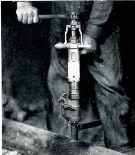
5. A Mueller E-4 drilling machine is used to drill into the gas main under pressure.
