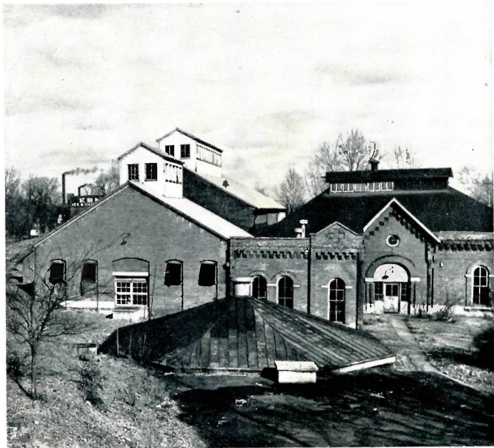
This is a view of Vincennes' filter house and pumping station (filter plant is at the left). Property was privately owned from 1886 until 1935, when it was acquired by the city itself.
