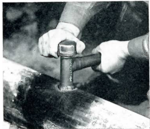
7. Completion cap is securely screwed on fitting, and the installation is complete.
