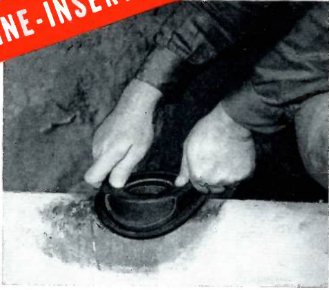
1. First step in the installation is to thoroughly clean the main before placing the gasket and saddle of the Mueller B gas tapping and inserting machine in position.
