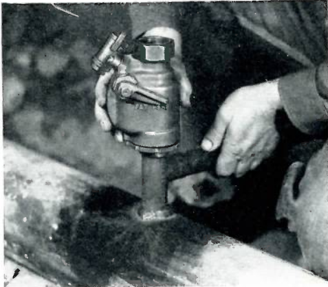
4. Control chamber (or Mueller gate valve) is securely attached to the welding tee.
