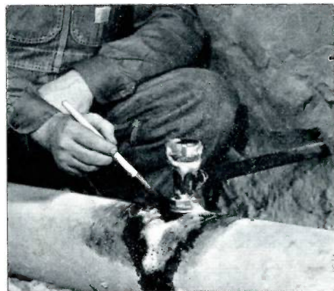
10. With the service line connected, the built-in valve is opened and the cast iron cap screwed on, completing the job except for testing under pressure with soapsuds.
