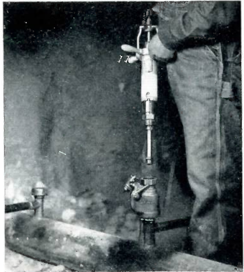
6. Bronze plug is inserted in tee by means of machine's inserting and extracting tool.
