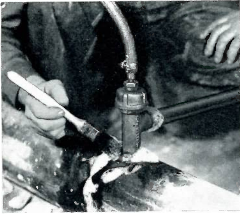
3. Test cap is screwed on fitting, air pressure applied, and welds tested with soapsuds.
