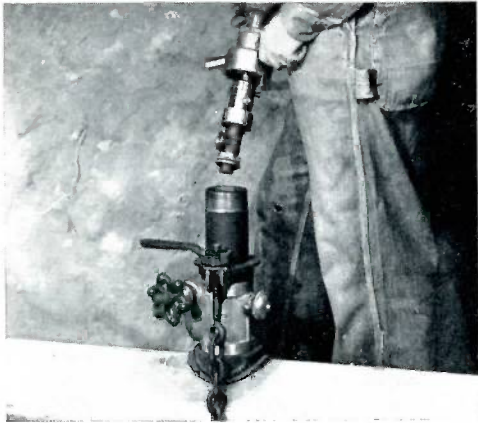
6. The cap and boring bar, which carries the screw plug and the tee, are placed on the machine, and the tee inserted in the drilled and tapped main without loss of gas.
