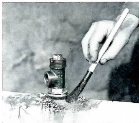
7. Chips from the drilling and tapping operation are carefully brushed away so as not to interfere with the copper-retained rubber gasket at the base of the service tee.
