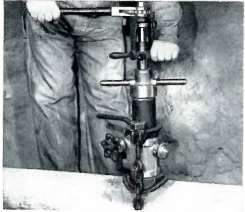
4. Using the Mueller B gas tapping and inserting machine, the main is drilled and tapped under pressure. Operator regulates amount of feed for tool with the feed yoke.
