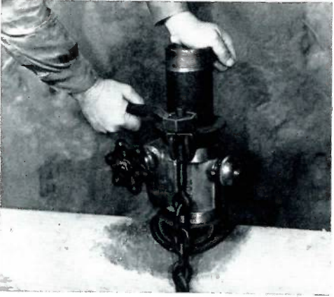
2. Lower portion of machine is placed on saddle and securely chained to the main. The machine should be drawn down solidly by evenly tightening both nuts on chain yoke.
