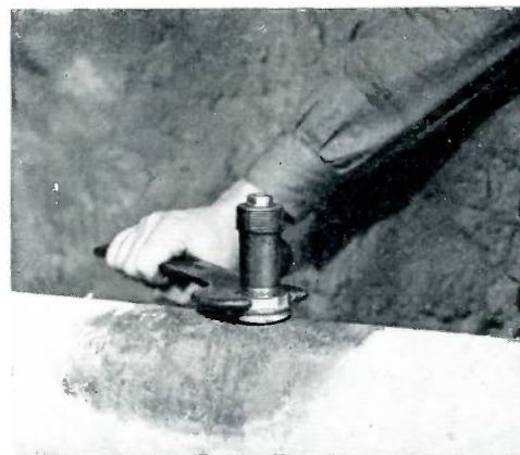
8. The tee is permanently tightened by hand. Tightening the compression nut forces the sealing ring against the surface of the pipe and the plain portion of the valve tee inlet.
