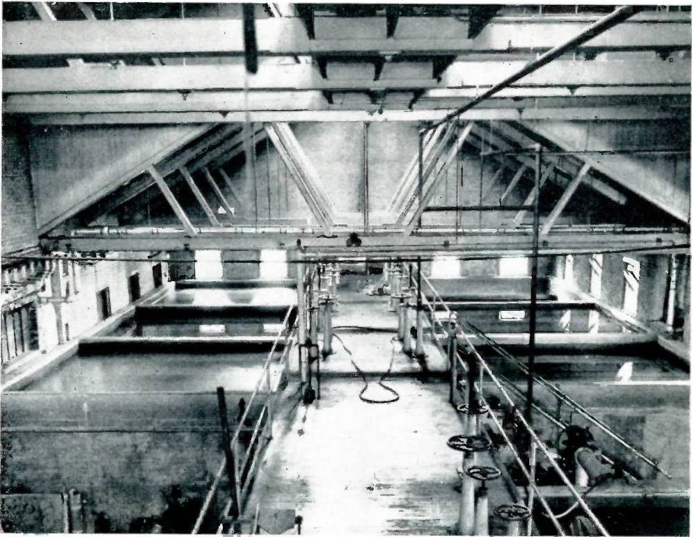
An interior view of a section of the filter house. The plant has nine filter beds, each with a capacity of 500,000 gallons. The main source of supply for the city is the Wabash River.
