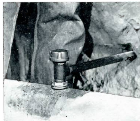
11. This photograph shows the completed installation. Gas to service line may be shut off at tee by removing the cap and closing built-in valve without further use of machine.
