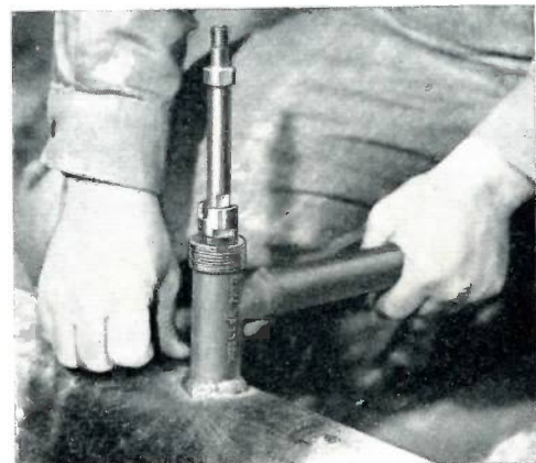
8. Inserting and extracting tool in position for removing plug for gas service shut-off.
