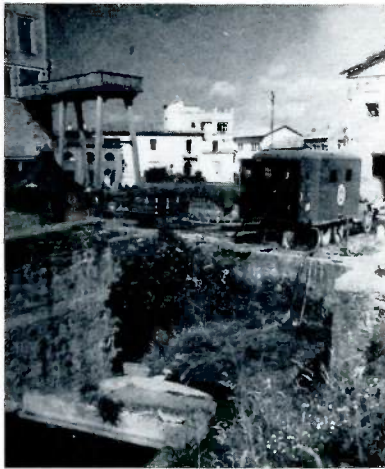
A company water point at Viterbo.
