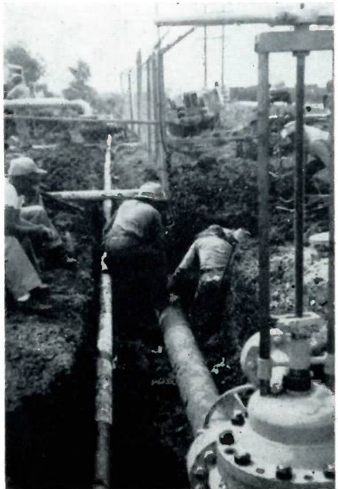
A 90 degree ell being installed in stopped off line.
