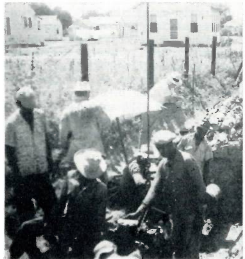
This view shows plug valve being installed in open section of the line.
