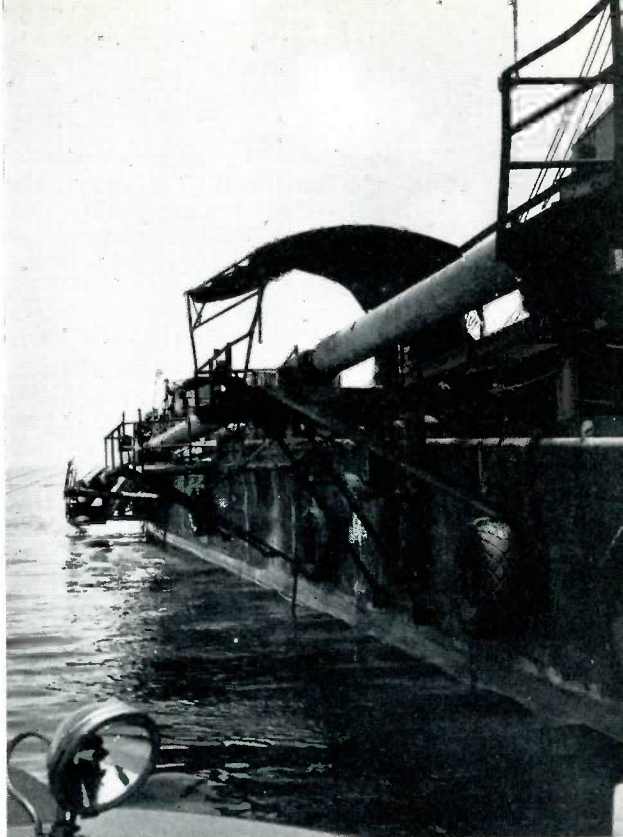
A 14-inch natural gas pipe line being laid in the Gulf of Mexico off the Louisiana shore.
