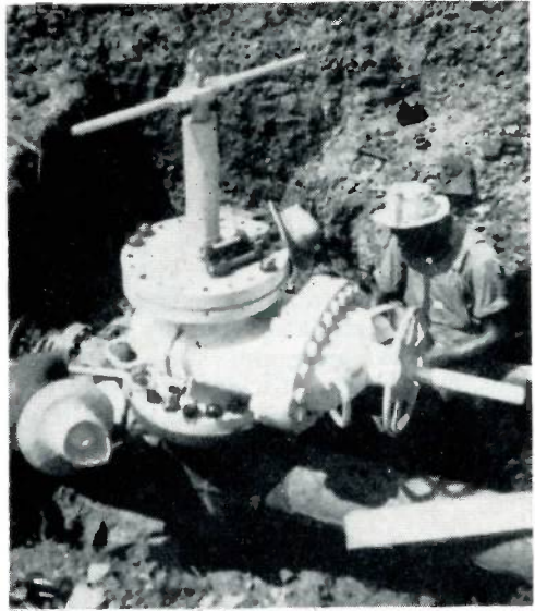
Mueller H-17445 completion machine assembled on line stopper fitting for insertion of the completion plug in the top of the fitting.
