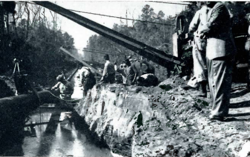
The line is placed into position.
