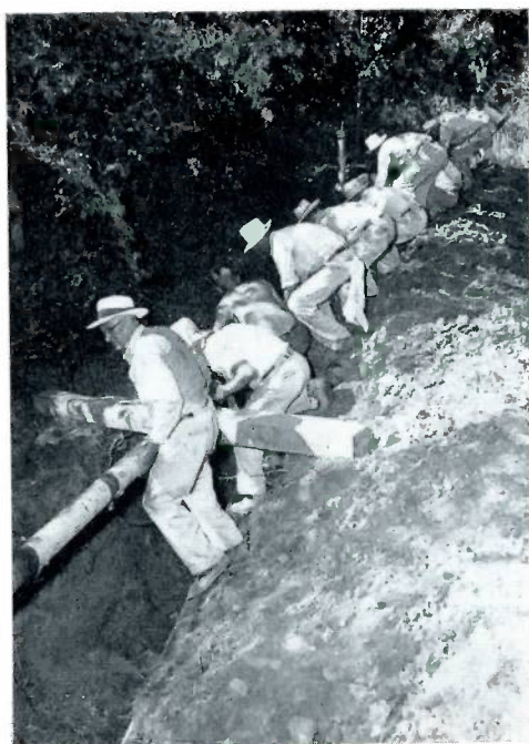
"E" Mainliners line up the new gas line before welding.
