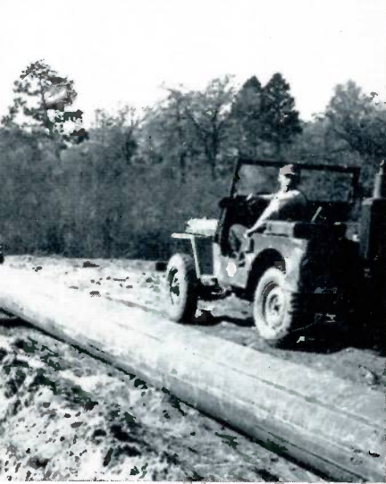
the transmission line.
