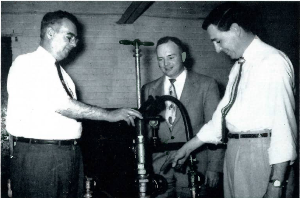
Assuming repairs have been made to the existing line, John Halvachs, left, General Division Superintendent, and Robert Jebavy, Gas Engineer, prepare to remove the machine. The boring bar brings up the stopper and Jack Leahy, Mueller Co. Sales Representative, points out that the gate valve must be closed before the machine is removed.
