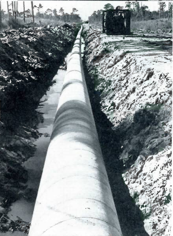
These "before-and-after" shots show the pipe lying alongside the ditch, and then show it wrapped and in place.
