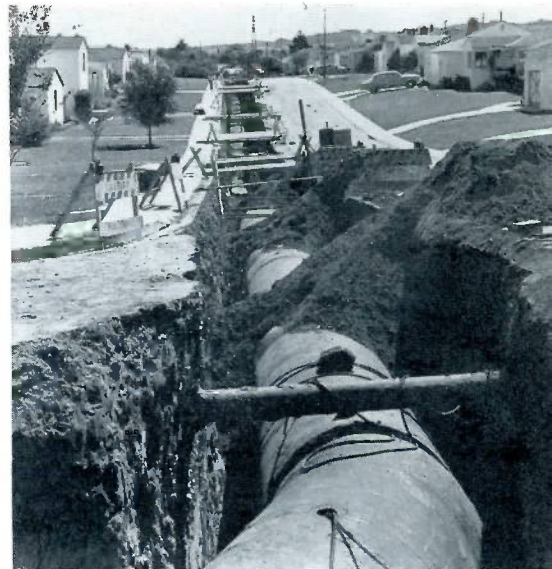
Above center: A 60-inch pipe on a 40-foot right-of-way traverses the back yards of a subdivision in South San Francisco. Above right: A 60-inch section of the Sunset Line snakes its way under a street in San Bruno.
