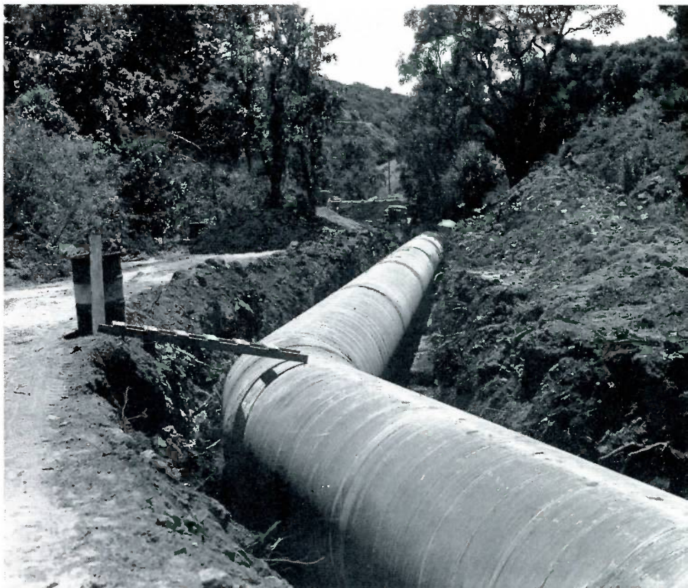
This section of 79-inch pipe is shown in place in the canyon below Crystal Springs Dam.
