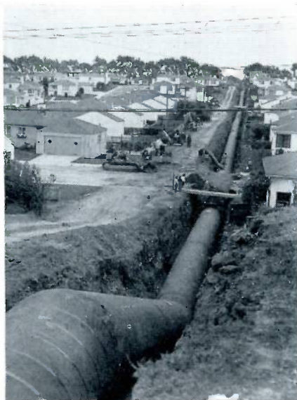
In the large photo at left, the 79-inch Sunset Supply Line is being laid in Hillsborough, Calif. The inset photo shows a 78-inch section of the same line. Above left: A 78-inch section of the Sunset line is ready to be covered.
