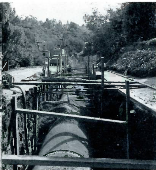
In the large photo at left, the 79-inch Sunset Supply Line is being laid in Hillsborough, Calif. The inset photo shows a 78-inch section of the same line. Above left: A 78-inch section of the Sunset line is ready to be covered.
