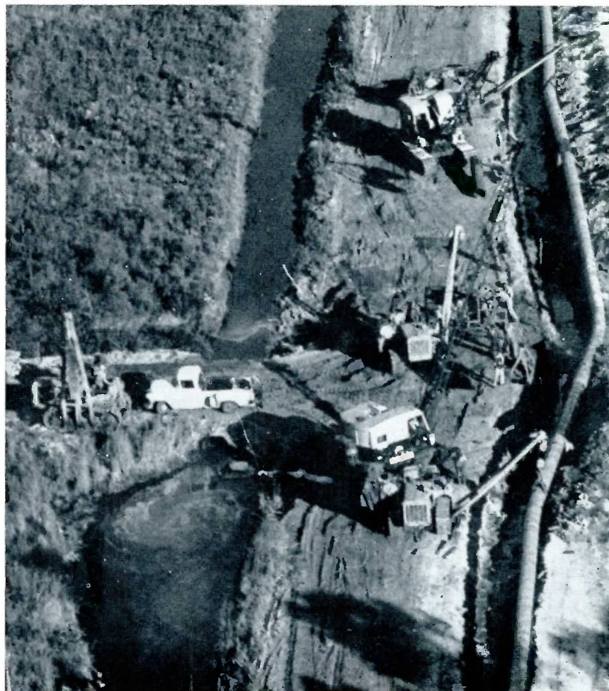
Giant cranes maneuver the lengths of pipe into position somewhere in Florida as the pipeline construction moves forward at a rapid pace.
