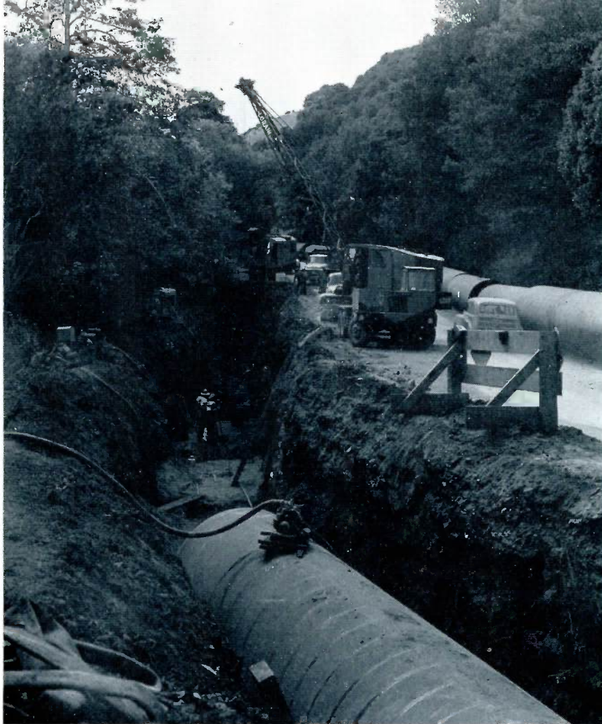
This photo shows a section of 79-inch pipe running alongside the state highway near Crystal Springs Dam. This is part of the Sunset Supply Line.
