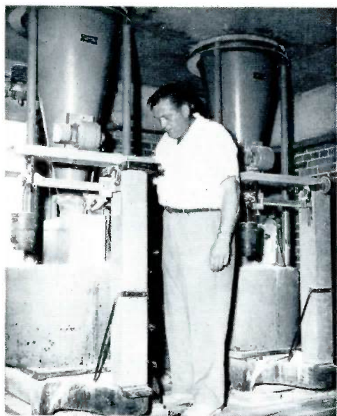
Superintendent Jason N. Daykin checks the flow of lime through the permutit dry chemical feeder. The chemical feeder hoppers above the feeders extend through the ceiling to the third floor where all chemicals are stored.
