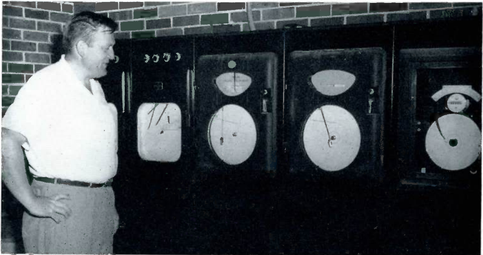
Mr. Daykin checks the control and instrument panel which is located directly behind the office and laboratory.
