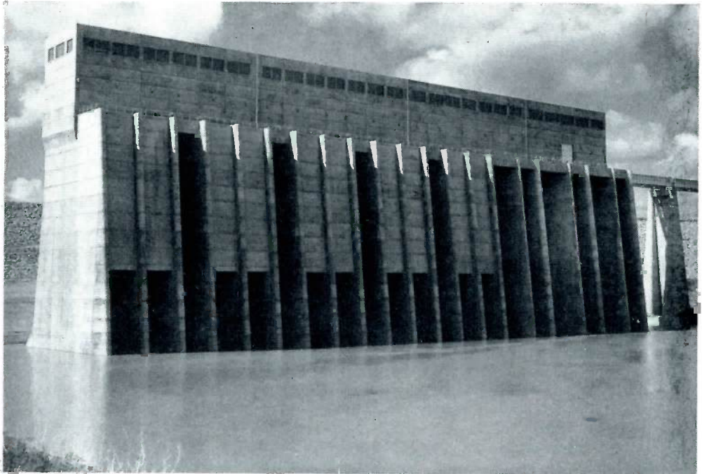
Exterior view of the giant intake structure, a 260 foot concrete shaft, housing the machinery for operating and controlling the flow through the tunnels.
