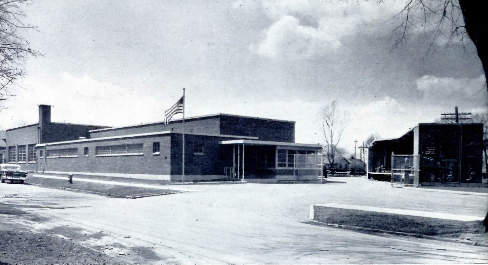
Pictured above is the Kemble Street Supply Center and Meter Shop of the Utica, New York, Board of Water Supply.
