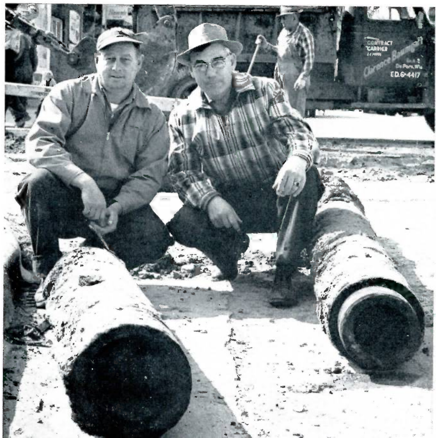
Anthony Van Remontel, a water department employee, and Superintendent LeMay, display the wooden mains, which are thought to have been in service 75 or 80 years.
