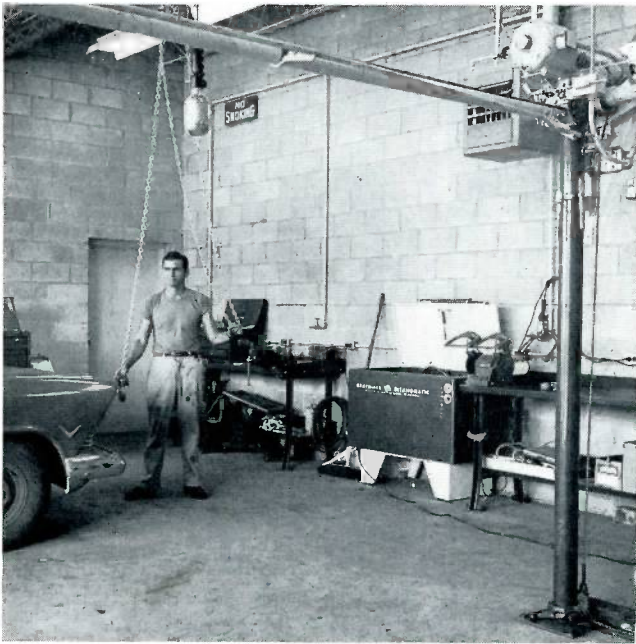
Allen L. Hyden, auto mechanic, works with valve refacing machine.
