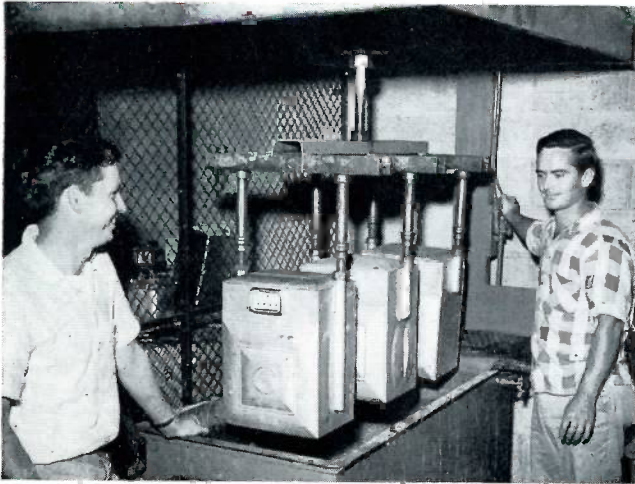
Tin meters go in stripping tank where chemical takes paint off for soldering. Left to right are H. H. Thomas, in charge during Foreman P. J. O'Neill's absence, and A. L. Eades
