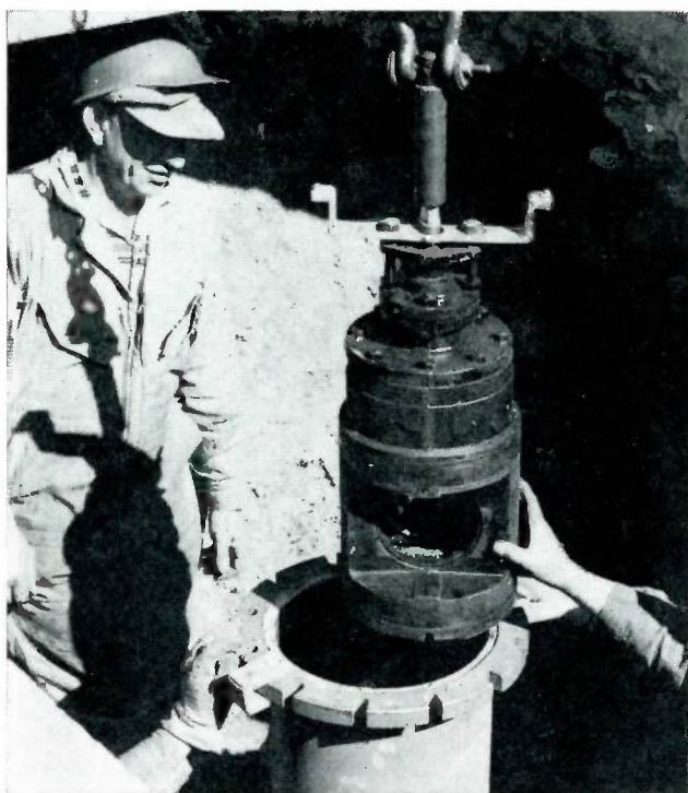
The gate valve assembly of the six-inch inserting valve is lowered (left) into the adapter and then into the valve body. The near finished valve is shown at the right. Once
