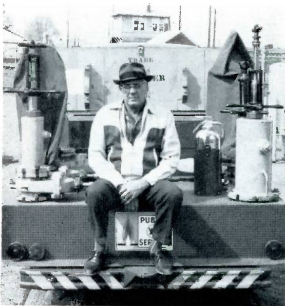
Superintendent Sanders sits between Mueller line stopping machines which are bolted to the bed of this truck which is used in the Kearney and Grand Island, Neb. area.
