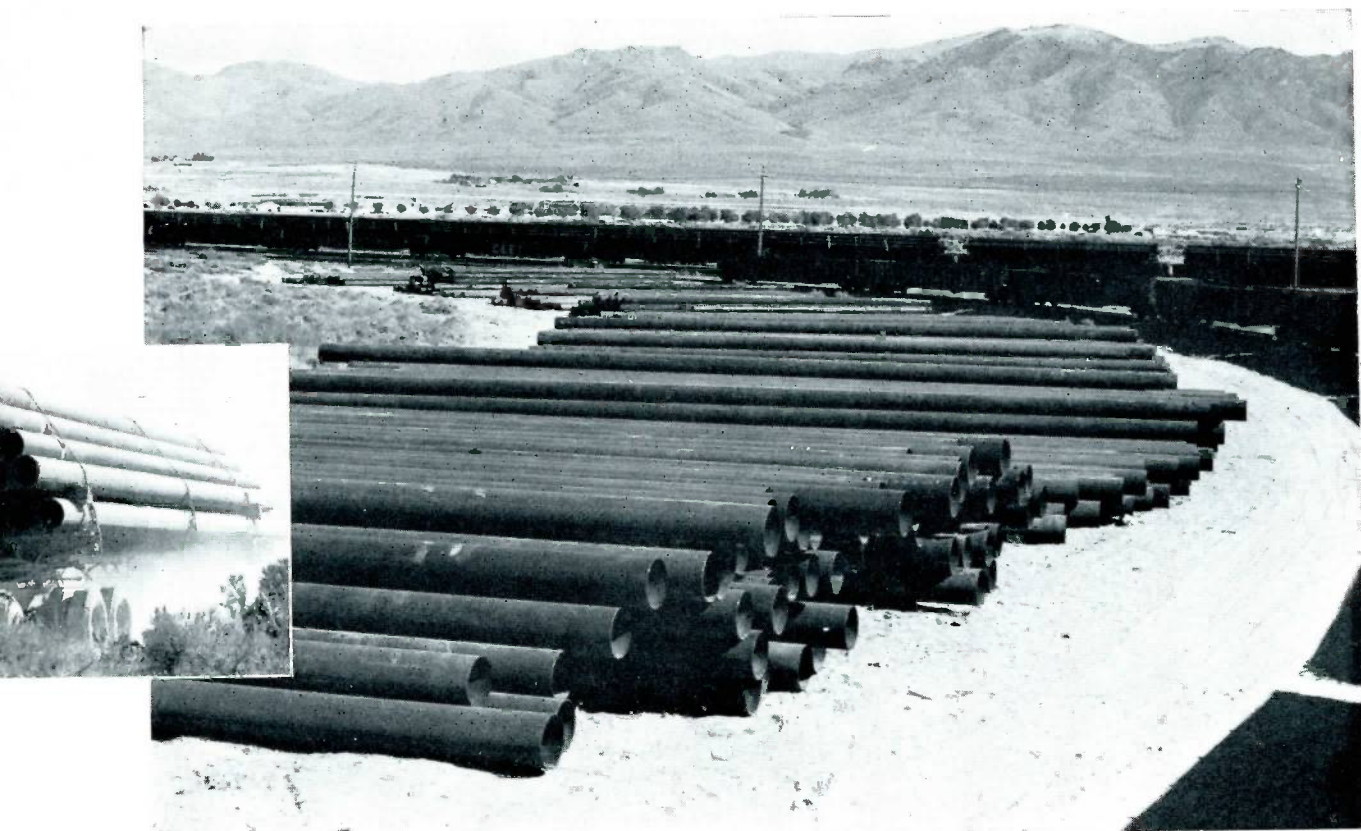
Rail cars stacked high with 16-inch steel pipe roll into Winnemucca siding where Wells Fargo trucks take the pipe to the site where the pipeline crews lineup the pipe preparatory to welding it together.
