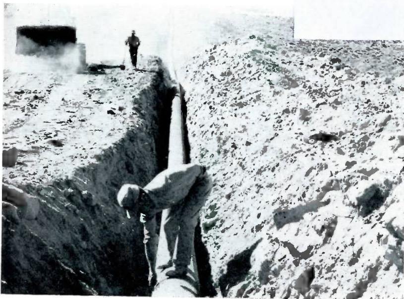
When the pipe is ready for lineup and welding, a clamp is drawn through it to the joint of the sections where it is held in place while a "stringer bead" weld is applied. This is followed by two more welds and then the joint is inspected by X-ray equipment. At the left a Nevada Northern Gas Company inspector follows the wrapping machine and marks any flaws in the protective cover.
