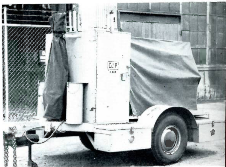
Protected by canvas, the Mueller machines stand poised for immediate use. The trailer can be hooked to any of the utility's service trucks and taken to a job site without more handling.
