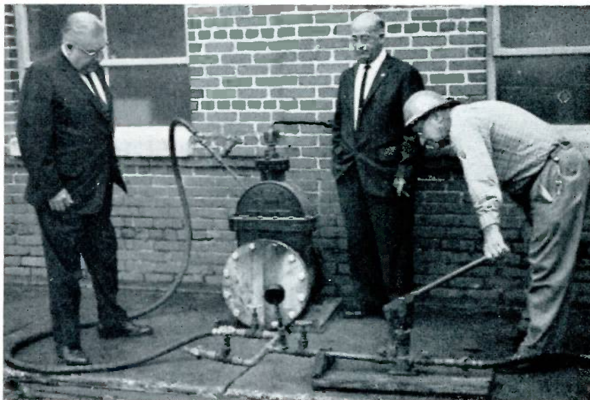
Giving a hydrostatic test to a Mueller 12-inch gate valve are, from left: J. P. Hawes, Assistant Superintendent of Distribution; A. Palermo, General Foreman, and O. L. Miller, valves foreman.
