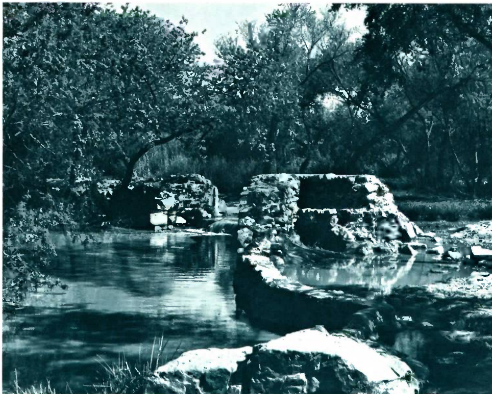
Spillway section of the Old Mission Dam and Flume which is an American Water Landmark in San Diego, California. The right side of the dam was washed away in 1916. (City of San Diego Photo)
