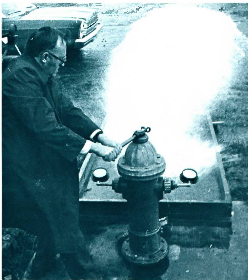
Donald E. Knibb, chief engineer for the Water and Sewer Department, operates a Mueller fire hydrant during a water volume test on a new 36 inch transmission line. Pressure gauges were placed on both capped 2½ inch hose connections and the 4½ inch pumper connection opened. Mr. Knibb said, "We did not know how much turbulence there might be in the hydrant head or how much difference we would observe between the two gauges. It developed that the pressures were even on both gauges and we recorded a peak residual pressure of 25 psi. Based on hydraulic tables of the Factory Insurance Association, we estimated that this would mean a flow of just over 2,700 gallons per minute." The static pressure on the line without the hydrant flowing was 69 psi.
