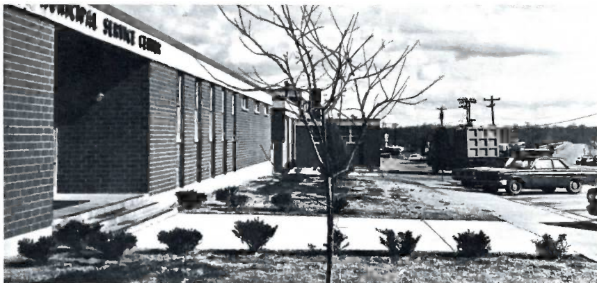
Inside and behind this administration building of the Municipal Service Center for the City of Greensboro are facilities for one of the most complete and functional operations of its type in the country.
