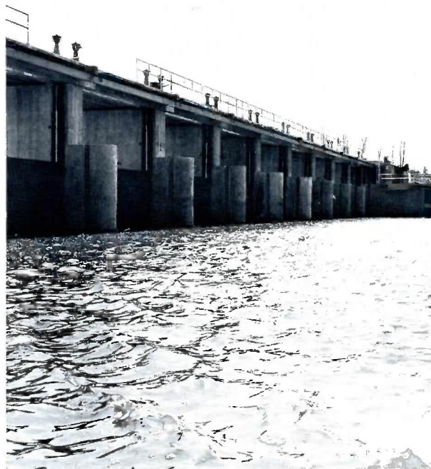
About 6,500,000,000 gallons of water for the City of Greensboro are stored in Lake Townsend which is formed by this 276 foot dam. The lake has a shore line of about 32 miles and an area of 1,440 acres.
