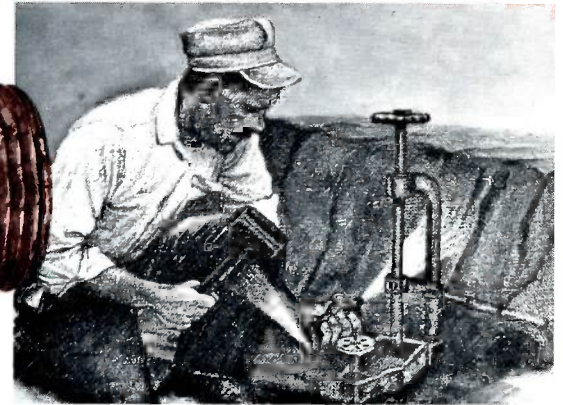
Service connections weren't always quick and easy to make. Prior to Mr. Mueller's tapping machine, workmen had to partially drill the main and then try to drive the corporation stop securely into place with a hammer. A dousing was the inevitable result.
