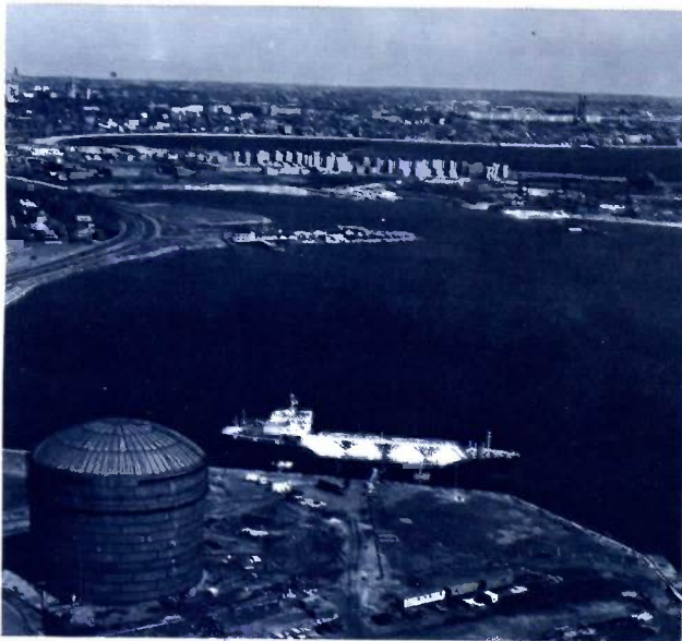
LNG arrives in the United States after a trans-ocean voyage. Massive investments have been made in facilities designed to handle the fuel when it is loaded and unloaded around the world. (Photo courtesy of Boston Gas Company.)
