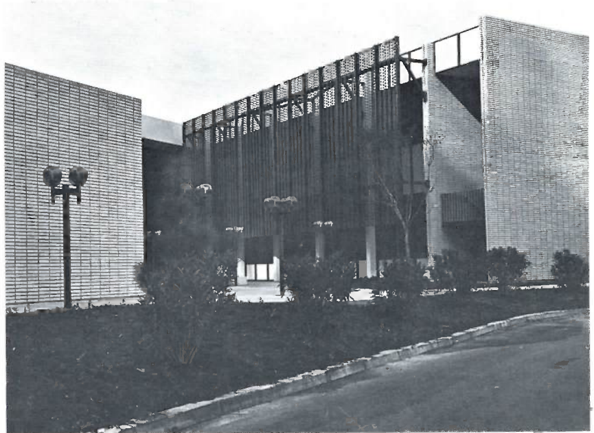
The east patio is located between the employee's lounge and the home service center in the left wing and the engineering and administrative offices on the right side of the building.
