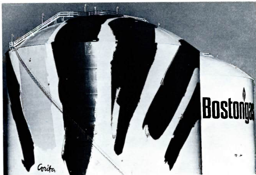
The rainbow design on Boston Gas Company's liquefied natural gas tank overlooking Dorchester Bay in Boston is acclaimed as the world's largest work of art since the Pyramids.
