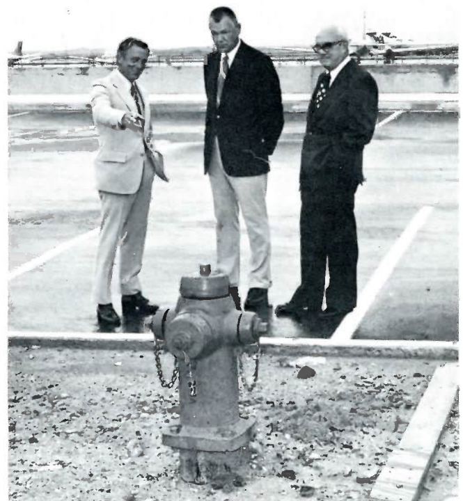
JACK CHILTON, Mueller Sales Representative from Dallas, points to one of the 75 MUELLER® Modern Improved Fire Hydrants installed at the DFW Airport. Shown with Jack is DFW's Supervisor of Utilities A. L. Utesch and R. D. Kitchen, Mueller Southwest District Sales Manager.
