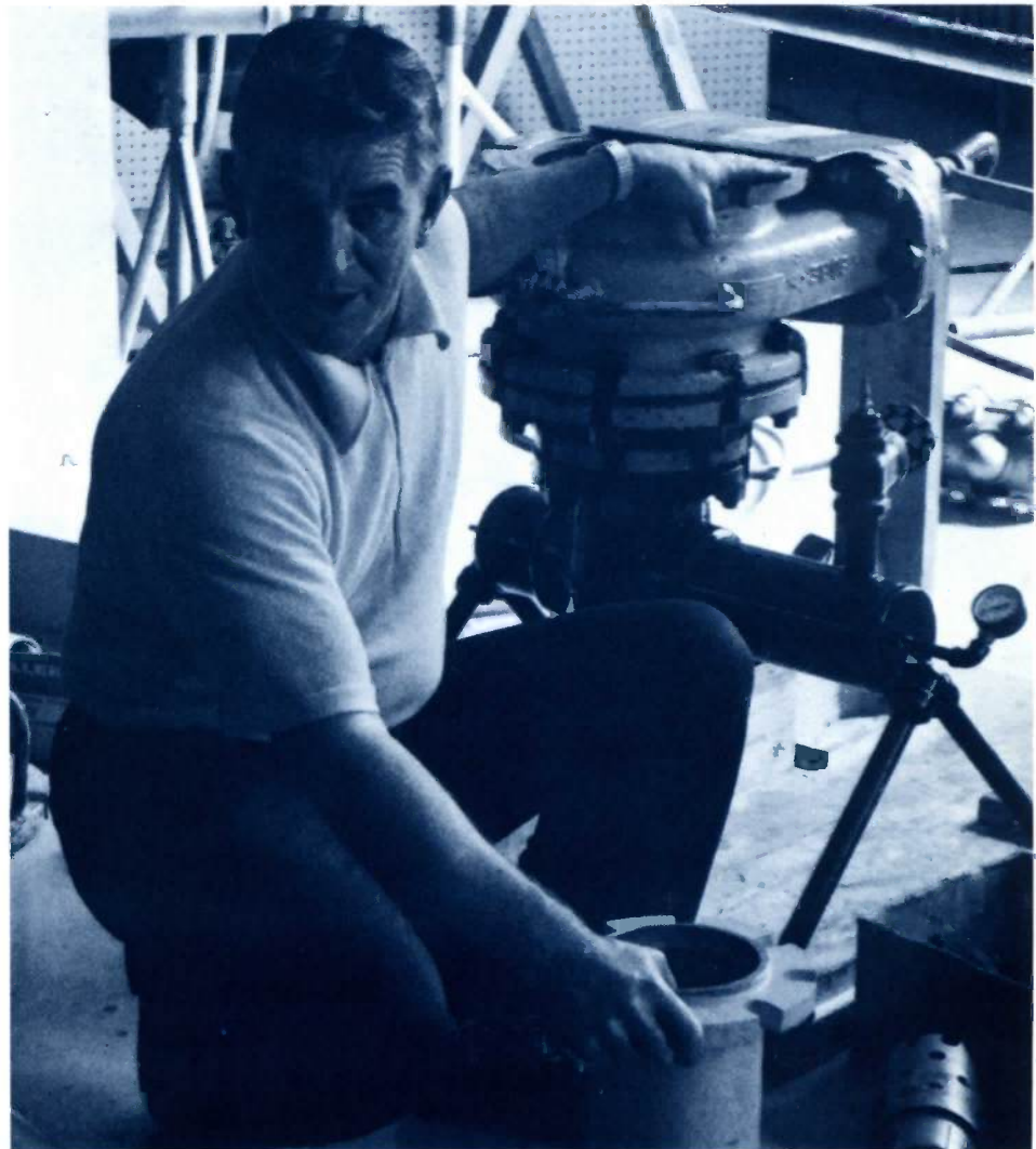
Bill Knorr explains the steps he will follow for a line stopper demonstration.
