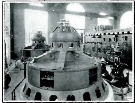
Interior view of the power house showing two 750-horsepower generators and switchboard.
