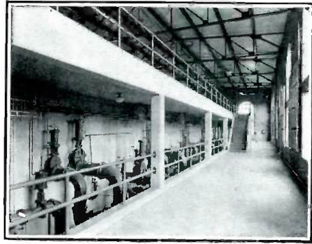
The pipe gallery on the first floor of the filter plant building at Spartanburg, N. C.
