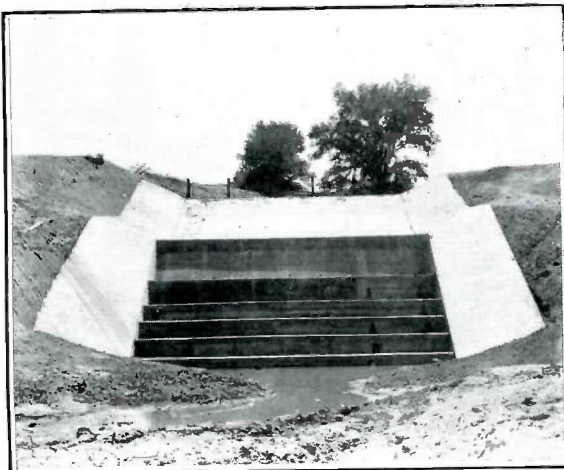
Showing spillway for releasing surplus water
