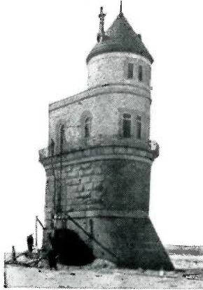
The West Intake at Chain of Rocks
