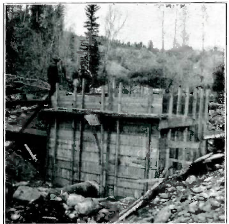
The intake well to the Main Line.
