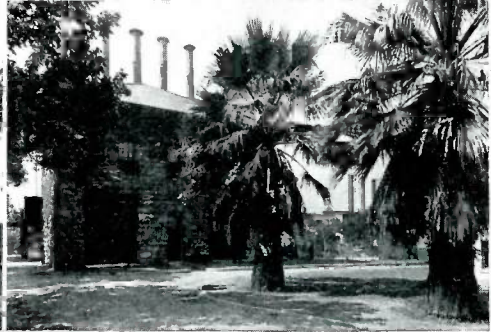
Market Street Station—the main pumping plant at San Antonio, Texas.
