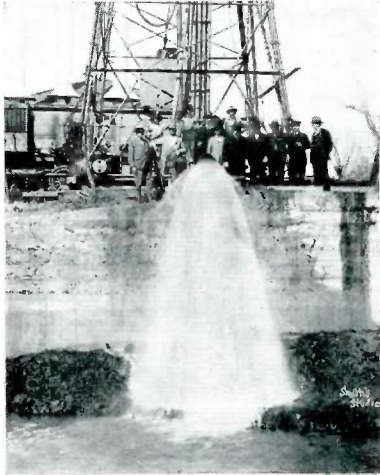
Twelve inch well brought in at the Market Street Station in 1923.
