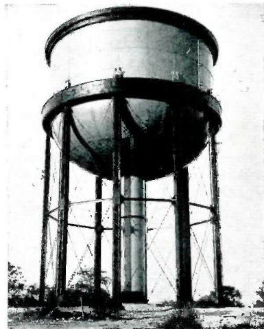
One million gallon elevated tank, north of Brackenridge Park.
