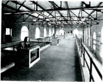
Interior of Spartanburg filter plant.
