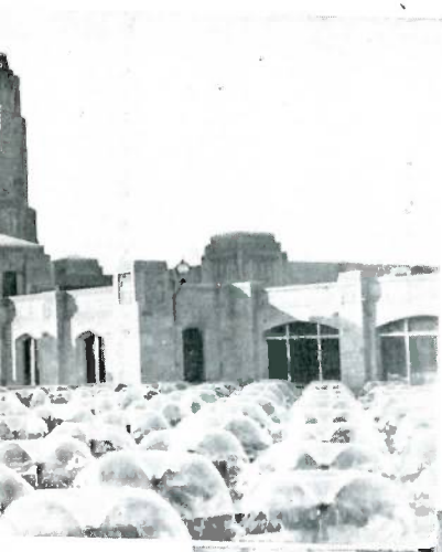
West Aeration Basin During Process of Operation
