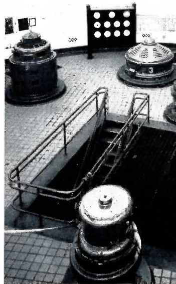
Below: Motor floor of low lift units equipped with vertical shaft
