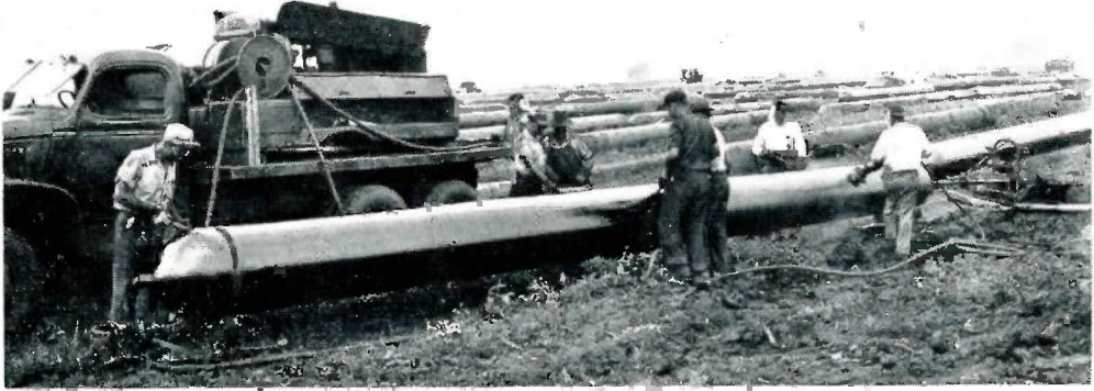
To prevent corrosion the pipe sections were coated with Bitumastic, a coal tar product, and wrapped with asbestos felt. Workmen here are shown cleaning and priming a pipe section preparatory to coating and wrapping. The work was done at the spot the pipe was to be installed in the ground, thus minimizing the handling of the sections after coating.
