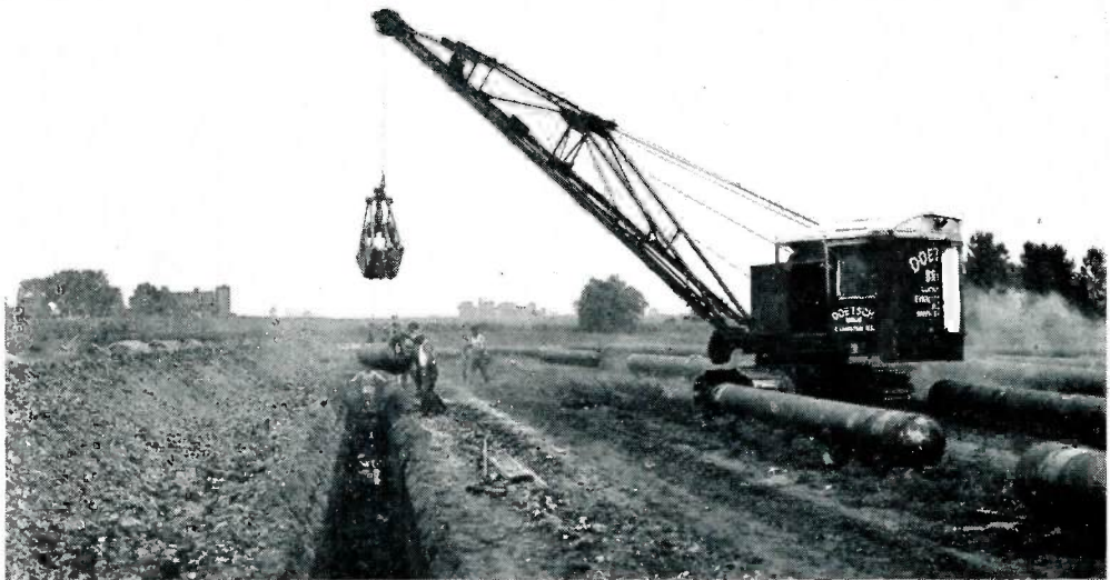
A 2½-ton pipe section is being lowered into a machine excavated trench, which is 36 inches wide. A special gauge was used to assure proper end-to-end spacing between sections, so that field cutting or bending of expansion bends would not be necessary. More than 15 miles of trenching were required for the 1,595 pipe sections in the 40-million C.F. storage field.
