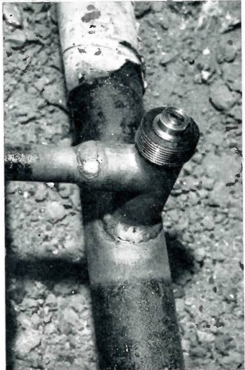
Right: This photograph shows the service tie-in at the main, using a Mueller H-10410-99003 Pin-Off Tee before the main is drilled. The tee is welded to the main and service lateral, forming a permanent, trouble-free connection.
