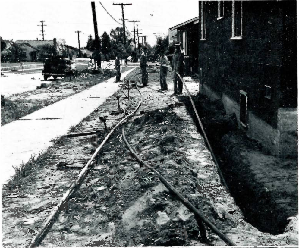
Above: Pipe sections are pushed through the bore to the gas main in the street. Natural deterioration and corrosion from moisture and other causes is prevented by wrapping and coating the pipe before it is placed underground.
