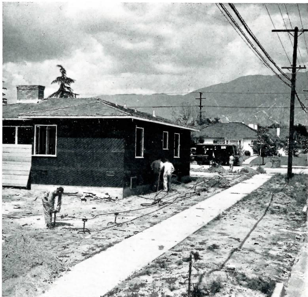
The workman in the foreground is pressure testing pipe, which has been welded in proper length and shape. In the background, servicemen are using an air motor to bore a tunnel to the main without damaging either the pavement or the sidewalk.
