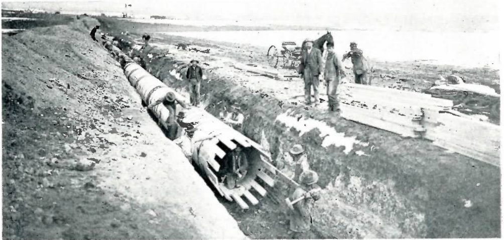
This 1911 photograph shows construction work on one of Denver's wood stave conduit lines, which delivered water from the South Platte River to Marston Lake, an impounding reservoir.
