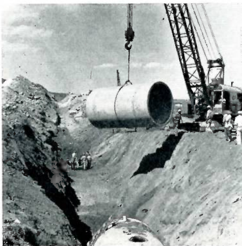
Denver's new 90-inch reinforced concrete pipeline will replace the old wood conduits.
