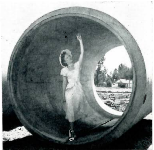
Each 16-foot length of the pipe weighed about 20 tons. First pipe was laid May 25, 1949.
