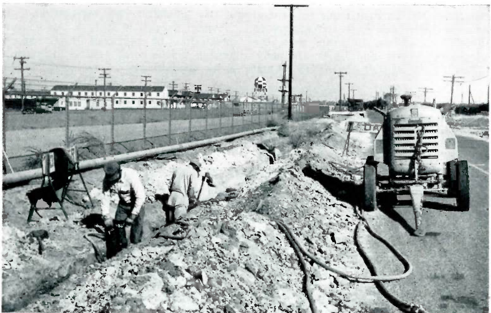
Due to its excellent flying weather, Arizona has several United States Air Force Bases within its borders. Located near Phoenix are Luke AFB and Williams AFB, both of which Public Service serves with natural gas. Above, company workmen install a main bringing gas service to Luke Field.
