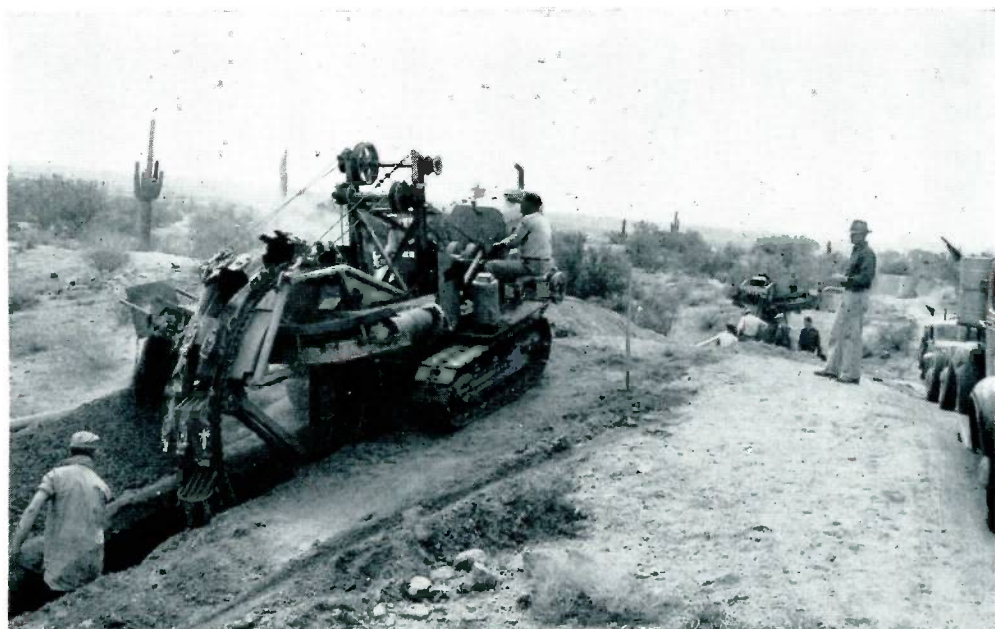
Although Arizona's population has increased fantastically in the past decade, there is still much desert land in the southern part of the state. Here, an Arizona Public Service crew trenches its way across the desert to bring natural gas service to another community.
