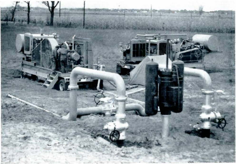
These three diesel engines are in the process of testing the first 400 mile portion of the American Louisiana Pipeline from Willow Run, Michigan, to Slaughter, Kentucky. A complete testing package consists of two low stage compressors and one high stage compressor. Nate Beal and Alfred Hickey of the American Louisiana Pipeline testing crew are examining the high stage compressor. (Authenticated News Photos)
