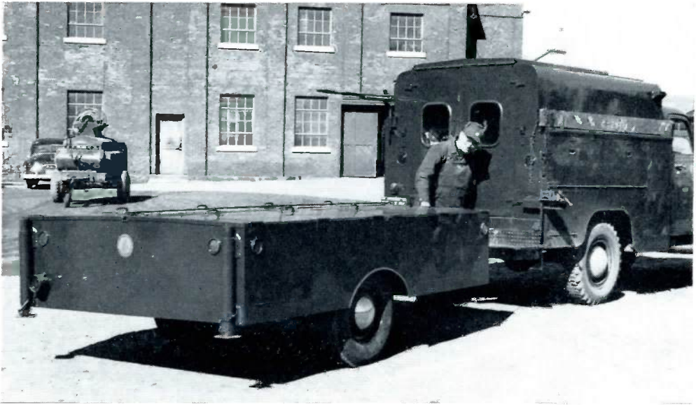
The truck is backed into the trailer carrying Mueller line stopper equipment. Keeping line stopper equipment ready for emergency use in this manner is proving to be very popular among several gas companies.
