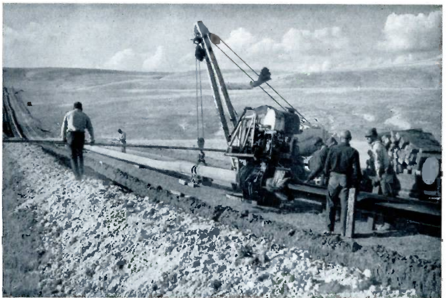
THE WARREN-BELFREY line construction at lower altitudes, indicating that the worst is over as the Montana Power crew nears its objective.
