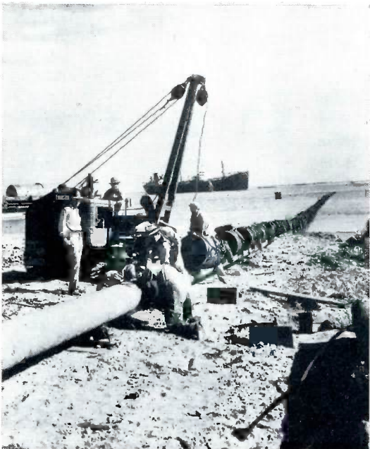
EVEN BAYS and rivers pose no obstacle to men who lay natural gas pipelines across the country. [Photo courtesy "Authenticated News"].
