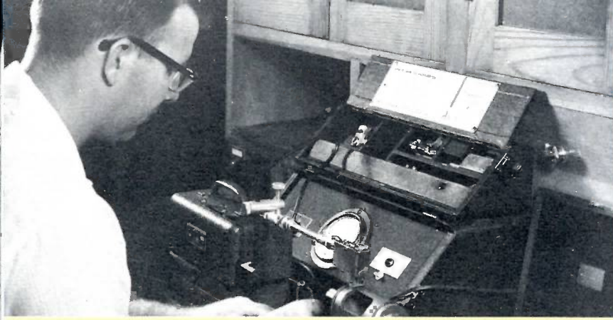
Surface smoothness and contour is revealed by a Profilmeter, a precise instrument that helps a corps of inspectors in their work.
