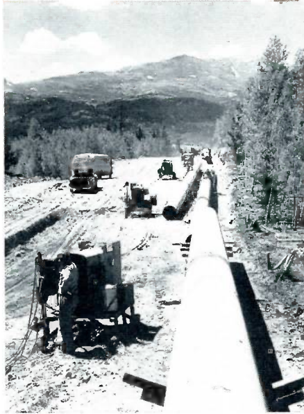
ON THE LEFT is a 20-inch iron main which feeds the northeast section of Colorado Springs. The inset again depicts the dexterity of these water department workmen as they lay lines through mountainous terrain in the vicinity of Colorado Springs. Above: the Lake George diversion dam, and two panoramic views to illustrate the length of the lines.
