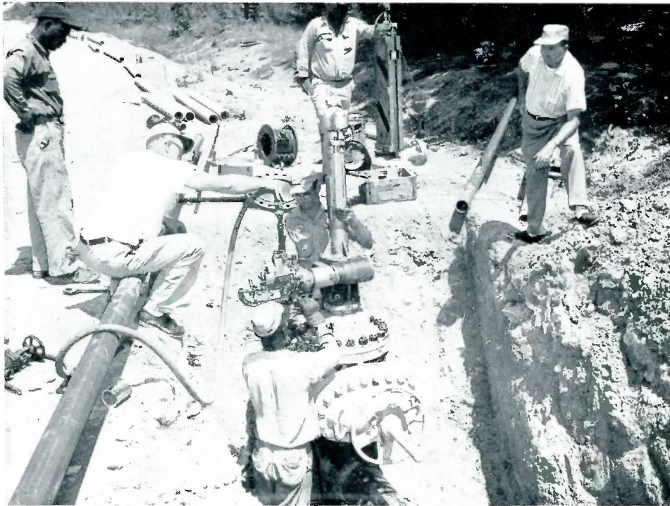
AT RIGHT, A. D. Parks, Southeast Sales Manager of Mueller Co. Seated is Jack Chepan, Mueller Service Engineer. This job involved lowering the transmission line of the Public Service Co. of North Carolina. Here the Mueller C-1 Tapping Machine goes into operation.
