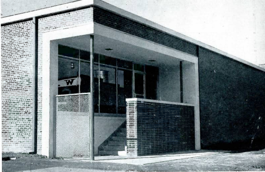
This is the main entrance of the new Gas Service Center. Completed early this year, the $100,000 building houses the meter shop, dispatching office, maintenance equipment, and several offices.
