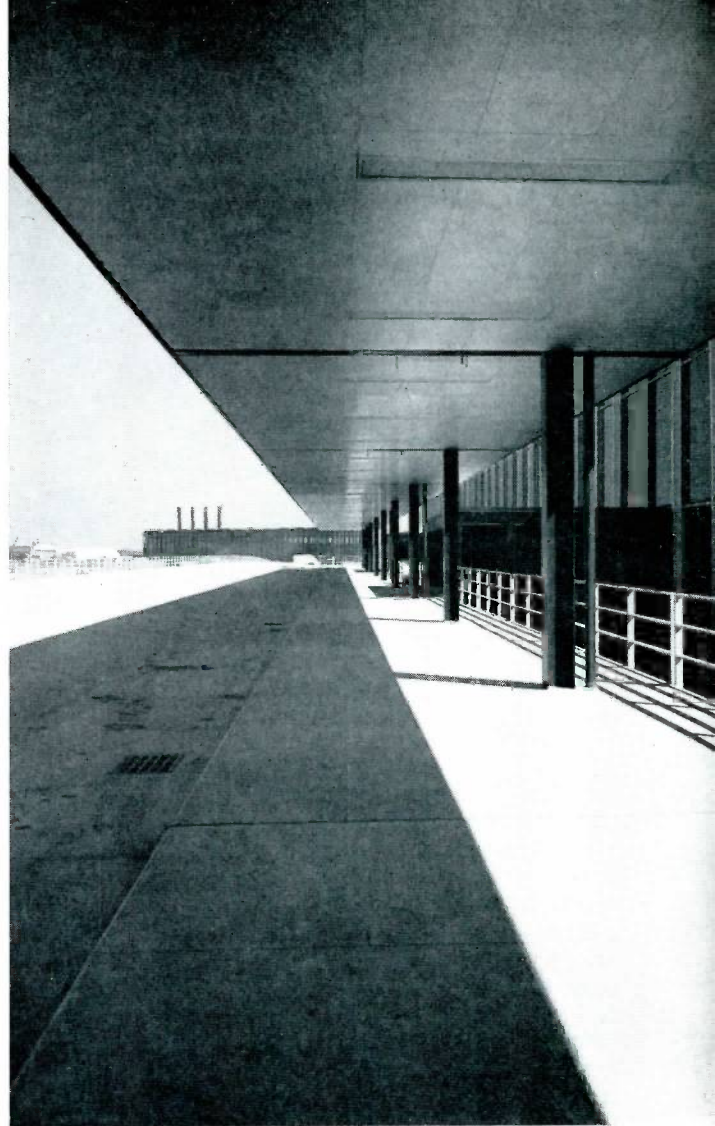
The vastness of the terminal buildings is illustrated by this view from the roadway near the entrance to the ticket offices.
