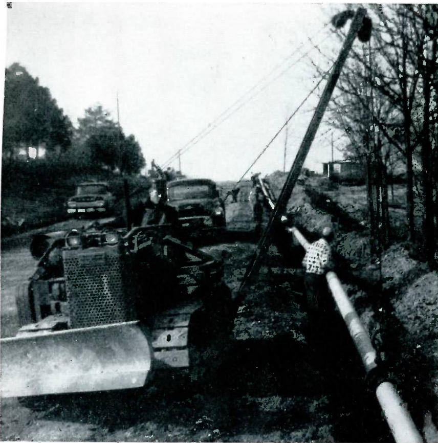
Workmen are laying a six-inch gas main to service the community which will have all of the comforts of big-city living. Most of the utilities are now in and construction will begin soon on the first 25 homes in the 2,800-acre development. Louisville Gas and Electric Co. will furnish gas for the city.
