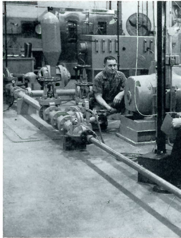
Checking a flow test is Project Engineer Lawrence Luckenbill (right) while Test Lab Operator Guy Pruett handles one of the controls. Beneath this
