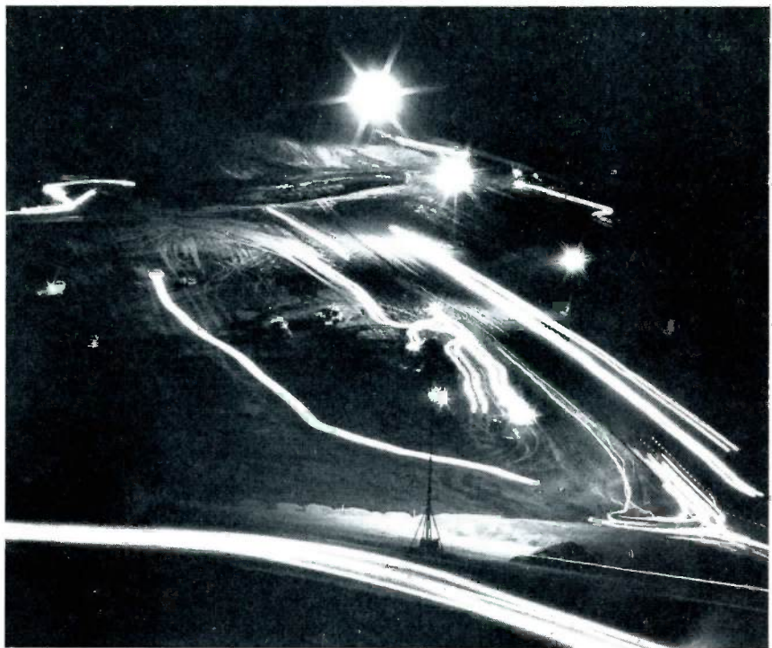
Headlights of giant earthmovers rumbling across the surface of Briones Dam near Orinda, Calif., produced this unusual night photograph. This dam, when complete, will produce a new reservoir for East Bay Municipal Utility District of Oakland, Calif.
