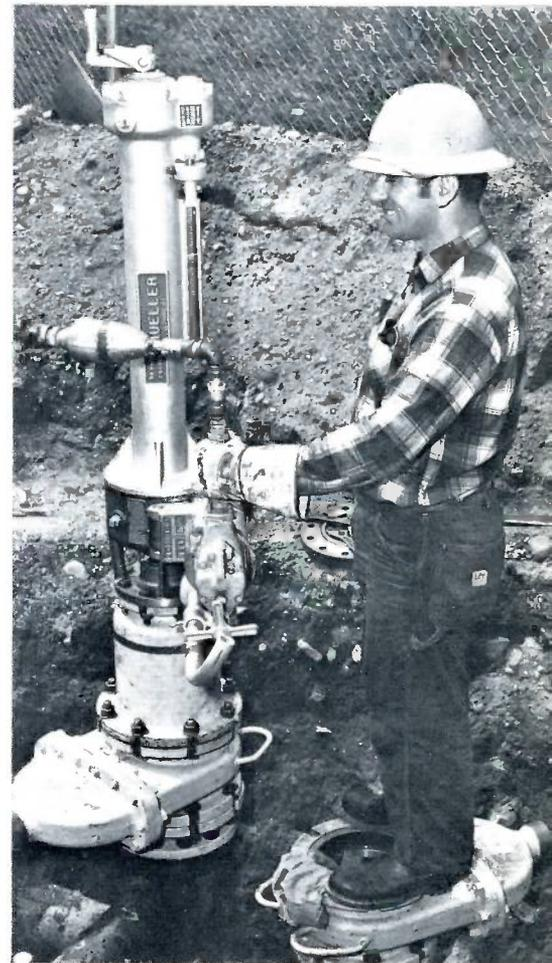
Operator for Consolidated Edison starts the air motor as he begins a cut with a Mueller machine.
