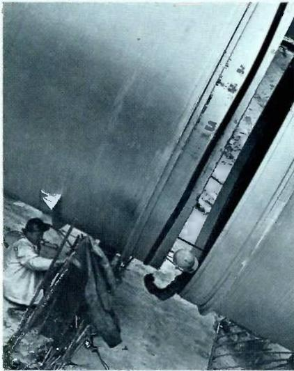
The 11½-foot-diameter pipe dwarfs workmen preparing to connect two lengths.
