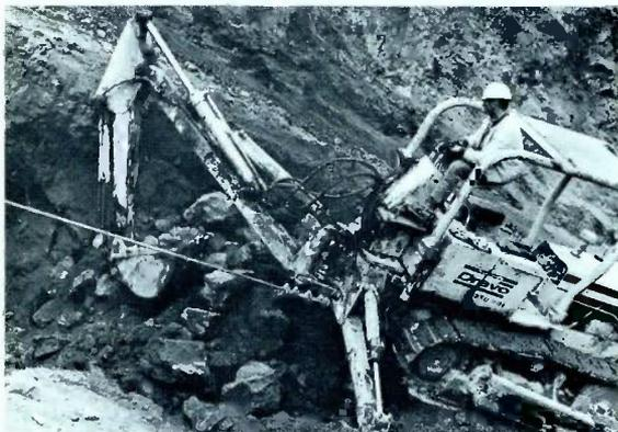
Backhoe digging foundations for concrete footings is held on steep hillside by a cable secured at the top of the slope.
