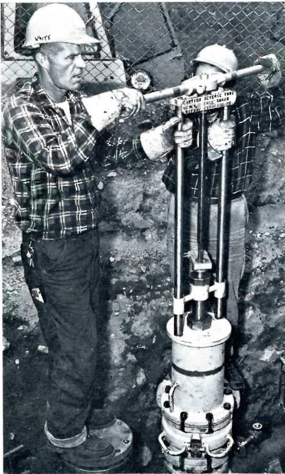
Drilling operations have been completed through both the flanged tee (left) and the line stopper fitting, and now the line stopping machine is in place as workmen expand the stopper.
