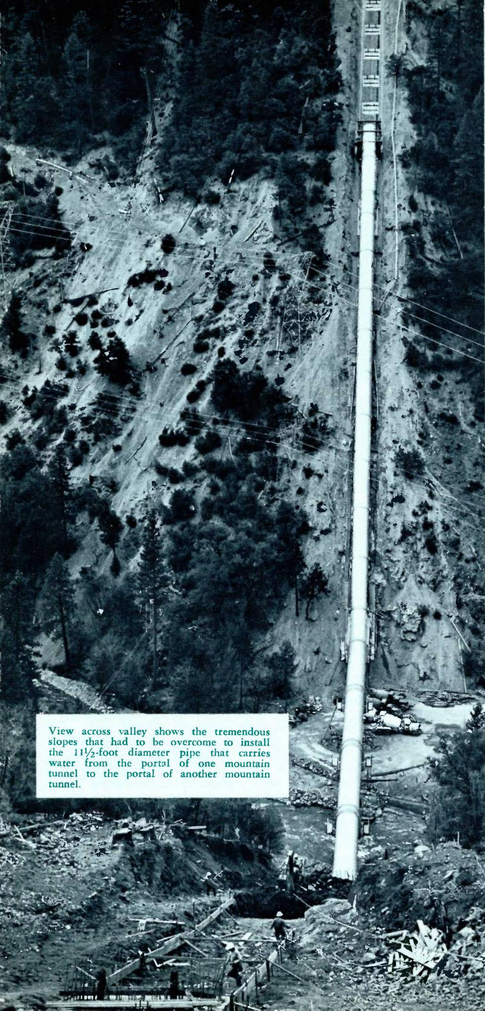
View across valley shows the tremendous slopes that had to be overcome to install the 11½-foot diameter pipe that carries water from the portal of one mountain tunnel to the portal of another mountain tunnel.
