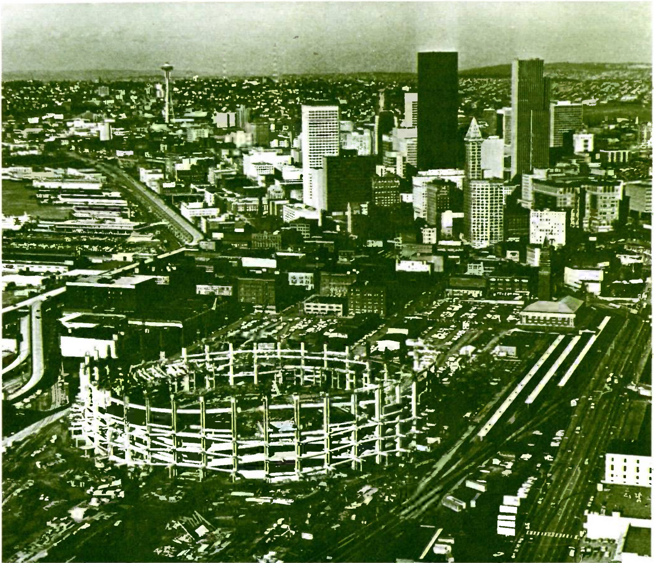
This aerial view of the new King County Stadium now under construction shows location within an area bounded by the Burlington Northern mainline railroad tracks, the recently renovated Pioneer Square district of Old Seattle and the city's historic waterfront.
