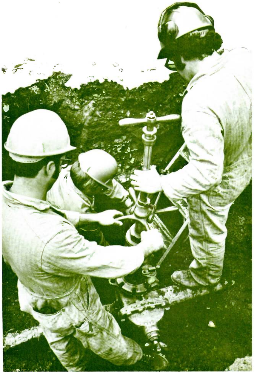
Mueller equipment is very much in evidence at the site of Seattle's King County domed stadium as Washington Natural Gas Company personnel prepare to extend 330 feet of 4-inch service to the facility's energy center using a Mueller line stopper fitting and the H-17235 stopping machine.
