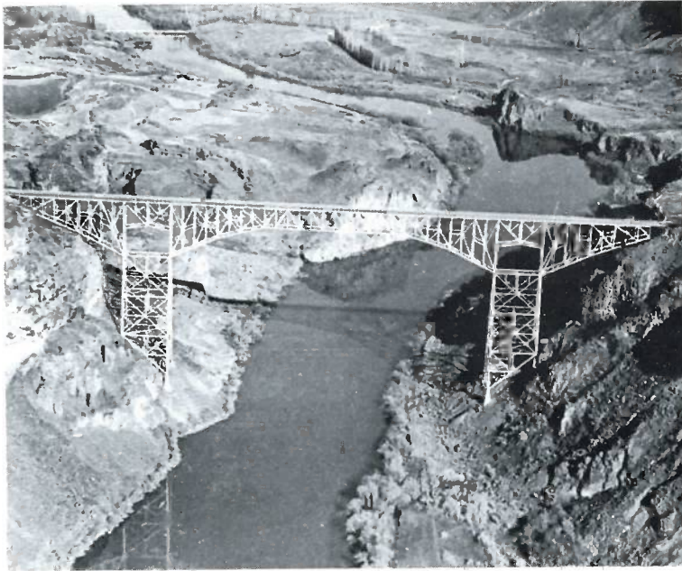
This is a panoramic view of the Snake River Canyon. In the foreground is the Perrine Memorial highway bridge at Twin Falls, Idaho. In the background can be seen the bridge carrying the Twin Falls lateral pipeline described in this story.
