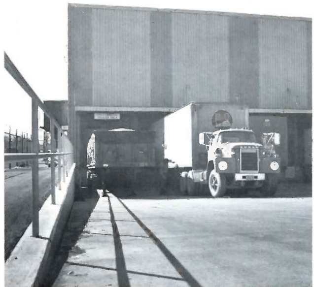
New shipping and receiving dock.
