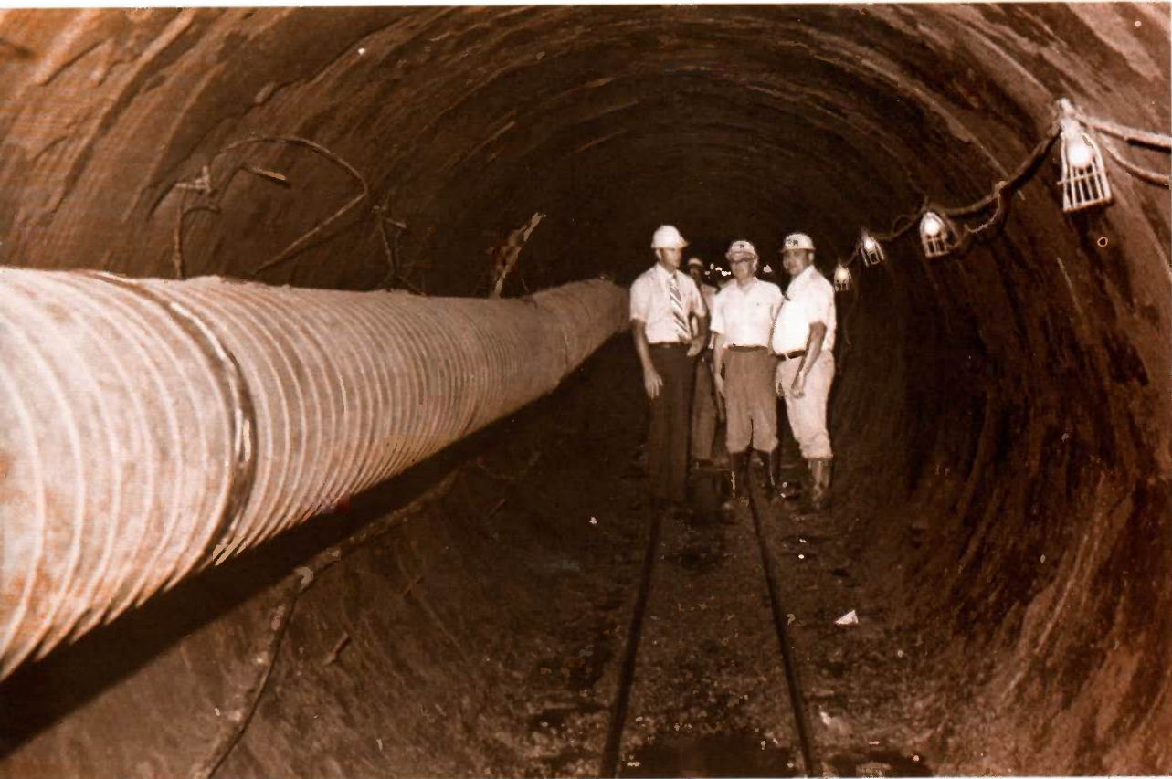
Standing in the marl tunnel far below the bottom of the Cooper River are Bob Maxwell, Mueller Representative, John R. Bettis, Commissioners of Public Works manager, and Steve Kinard, assistant manager.
