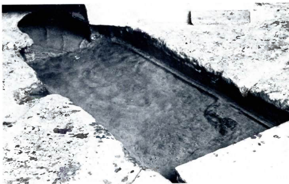
Where the Romans conquered, they took their knowledge with them. This masonry sluiceway conducted water into the pools at Bath, England.
