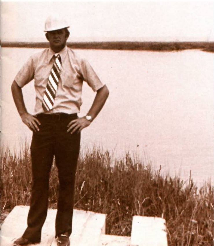
Behind Mueller Sales Representative Bob Maxwell, the Cooper River flows near Charleston, South Carolina. Amoco Chemical Corp's. new water tunnel lies 55 feet below the river channel.
