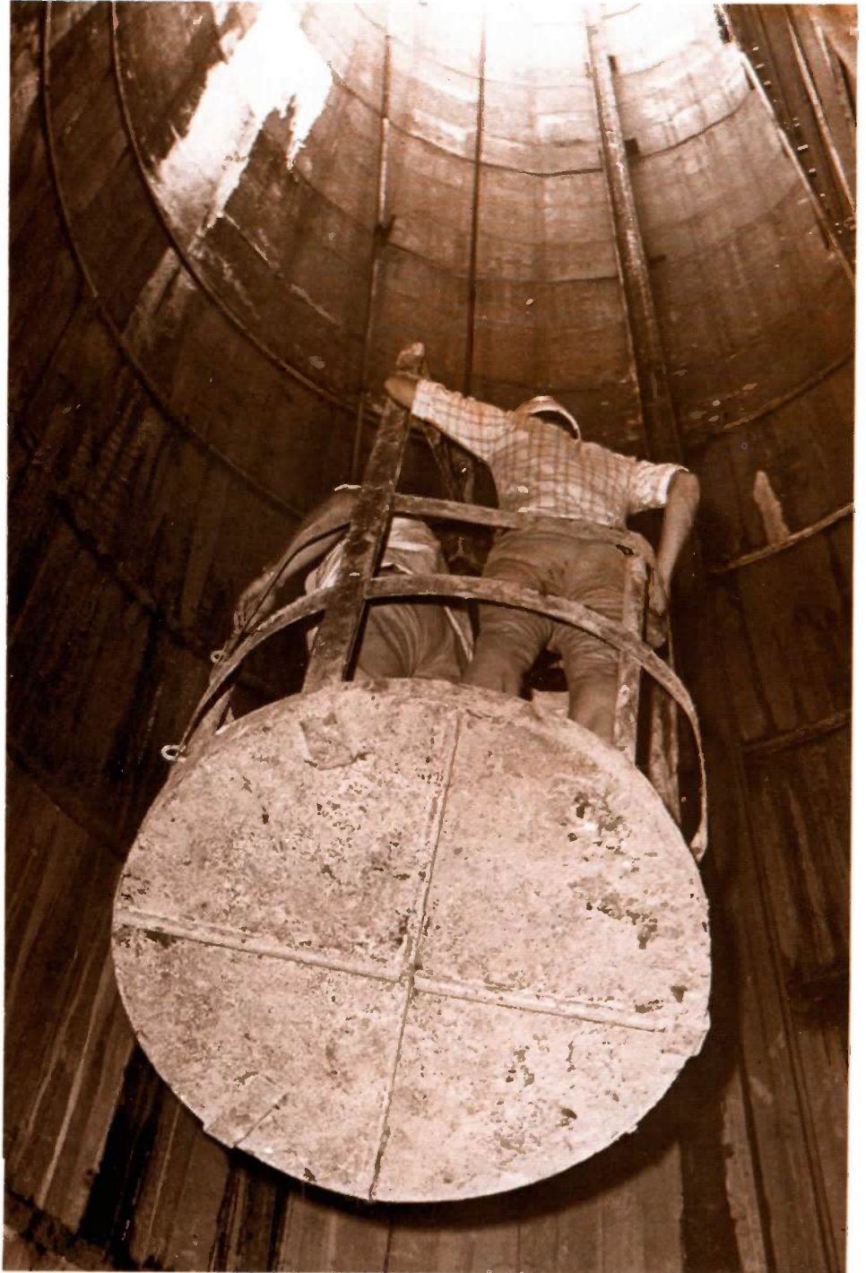
Having to go down the access shaft to the tunnel below, involves a ride in a cage lift suspended at the end of a cable.
