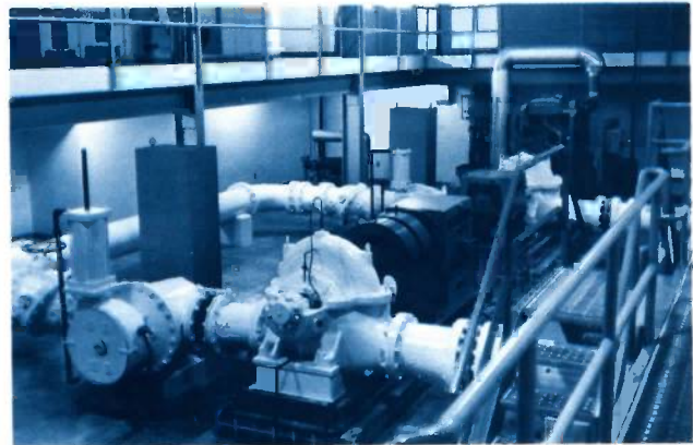
In the pumping room of one of the remote stations, the large pumps hum steadily as they help move the 46 million gallons that flow through the entire system during an average day.
