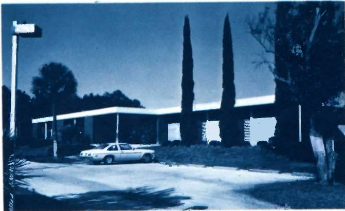
All 8 of the remote stations, like this one, may be operated on site if need be, but are normally controlled through the computerized control console in the main plant.
