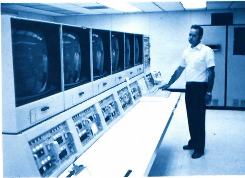
In the central control room — heart of the computerized system — John Banks monitors all of the vital signs (rates, pressures, levels, etc.) of the entire water operation. All of the remote pumping stations can be controlled from this room. This computerized control console, installed in 1973, was one of the first of its kind in the nation.
