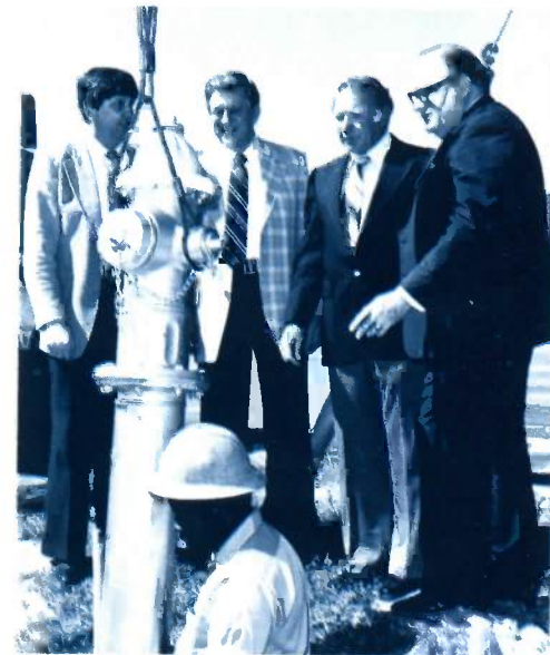
Another familiar sight in Orlando — the installation of a Mueller Centurion® Fire Hydrant. Watching the hydrant installation are, from left to right: Ted Pope, Manager of the Water Department; Bob Ott, General Sales Manager of Mueller Co.; Sam Parker, Mueller Co. Sales Representative for the Orlando area; and Curt Stanton, Executive Vice-President of the Orlando Utilities Commission.
