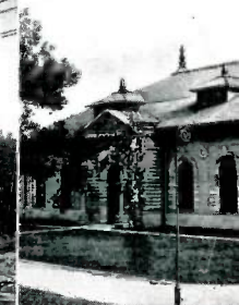
Ross Pumping Station which delivers adjacent filter plant. It was partially rehabilitated. It is an excellent emergency pumping station. The emergency conditions turbine driven centrifugal pumps driven by vertical steam boilers of 400 pounds.
