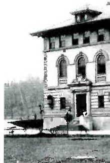
The Administration Building, Filtration Plant located east of the downtown section, chemical and bacteriological laboratory located in town.
