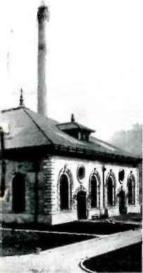
This is the low lift station for all river water to the city. In 1927-29 this station was replaced at a cost of $928,939. A sample of a high duty major equipment includes a new suction intake constructed under at a cost of $387,465; two 100 M.G.D. and one 50 M.G.D. steam engines; also one 50 M.G.D. and one 35 M.G.D. centrifugal pumps. The steam plant consists of two 600 H.P. sterling type steam pressure and 6 smaller boilers used only as reserve equipment.
