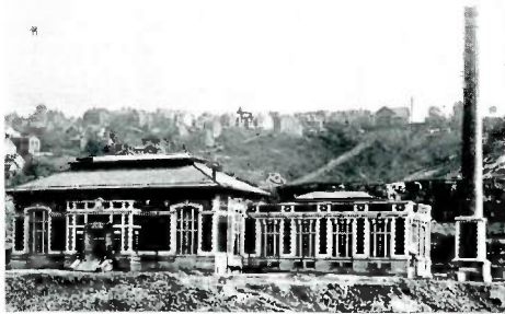
Mission Pumping Station, a secondary pumping station completed in 1912. Contains two 7 M.G.D. Vertical Triplex pumps and two 325 H.P. Boilers.
