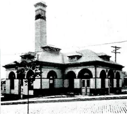
Lincoln Pumping station completed in 1895. A small secondary station containing two 1.1 M.G.D. electric motor driven pumps.
