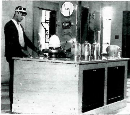
Master Control Table located in lobby.
