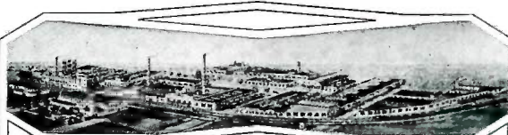
MAIN PLANT Decatur, Ill.
