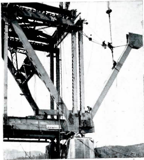
Riding bronchos is in line with a Merry-go-round compared to these fearless workers straddling ropes and wires while handling tons of iron 300 feet above ground.
