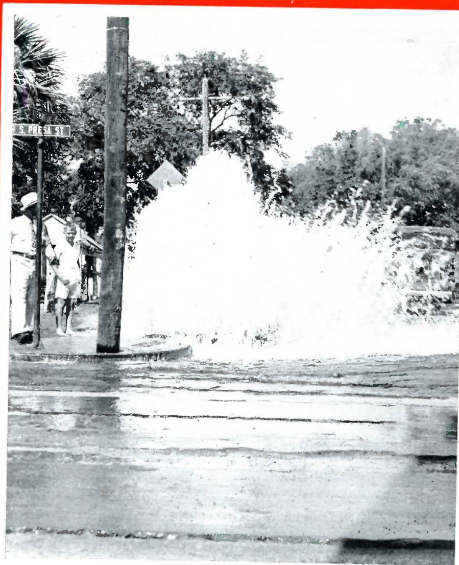
BURSTING MAIN WITH WATER OUT OF CONTROL
