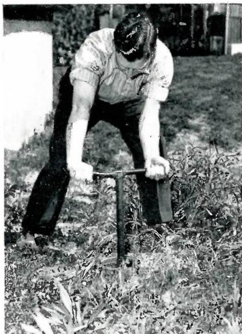
*Valve and valve box maintenance also will pay dividends. Periodic operation of valves prevents them from becoming so encrusted that they will not operate. Inspections may also show valve boxes paved over and valves not fully opened.*
