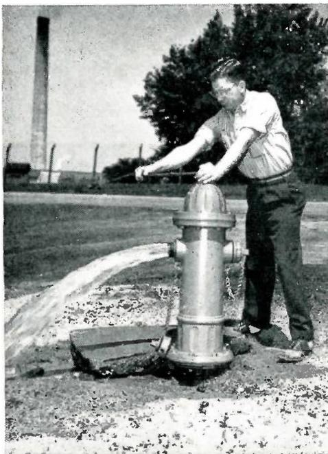
3 *Operating the hydrant from time to time serves to oil working parts automatically, offers a check on whether drain openings are clear, and determines whether or not the hydrant is in first-class shape.*
