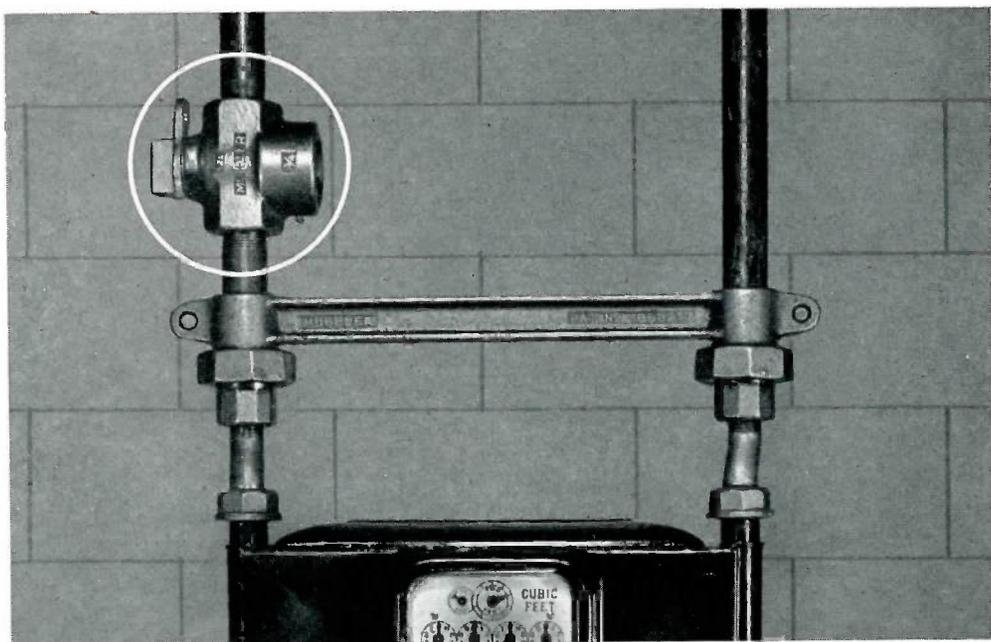
*The H-11112 lock wing gas meter stop, enclosed in white circle upper left, is shown as it appears in a typical meter installation. Its tamper-proof design and solid construction are features which are not available in any other make of gas meter stop. The individually ground and lapped key cannot be removed from the iron body without destroying the stop.*
