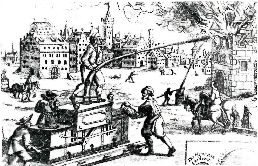
Modern pumpers apparently have little advantage over these hand-operated pumps of the seventeenth century, if the imagination of the artist can be trusted. This drawing, made in 1662, shows two models, the large, skid-mounted pump and the small, portable size. Note the barrels of water being brought up on horse-drawn skids to replenish the supply.
