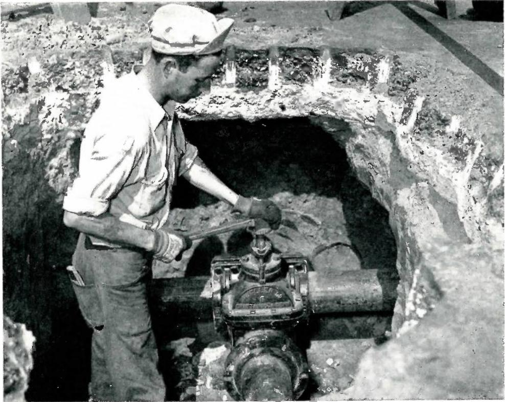
*Helper E. L. Moore opens the 6-inch tapping valve before the ditch was backfilled. A 6x4 reducer was used between the Mueller tapping valve and the cross shown below.*
