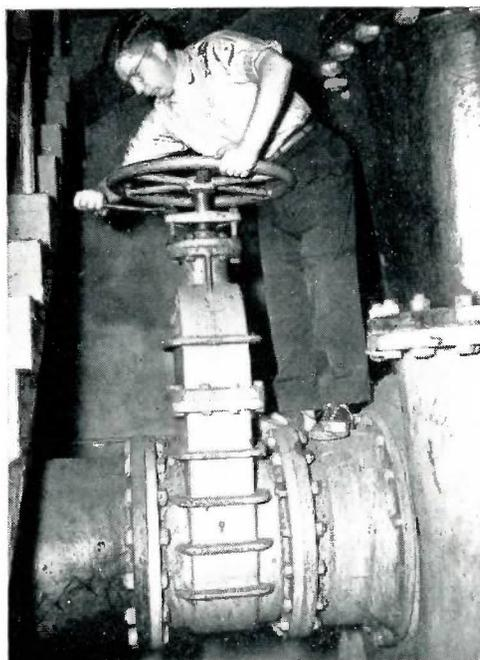
*Lubricate valves and tighten packing gland nuts, if required, on inspections. Preventive maintenance by periodic inspection and operation will rid water utilities of "one very large and painful headache," author says from experience.*
