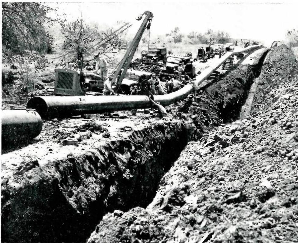
*A delay of two years in construction of the 405-mile gas pipe line was eliminated when Cities Service Gas Company purchased Steel plate at the mill, had it fabricated into pipe at another mill. Forty-foot joints of pipe are welded into lengths between one-fourth and one-half mile in length, depending upon topography, set in the ditch and covered.*
