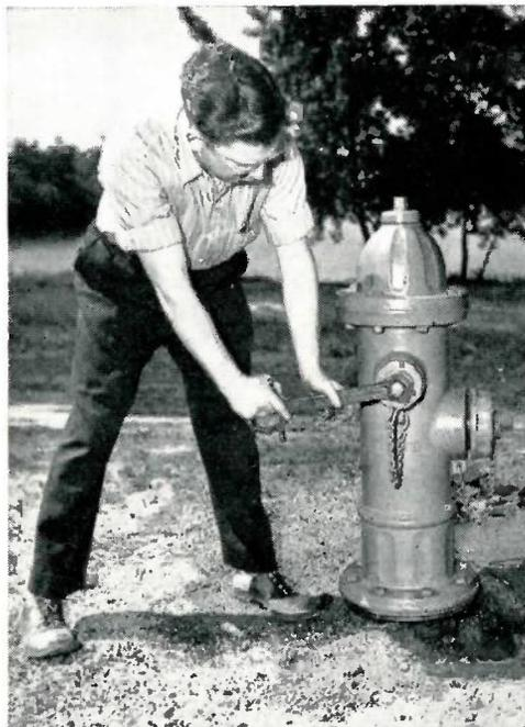
2 *Inspections also will determine whether nozzle caps are stuck, lost or off. Use a regular hydrant wrench to prevent mutilation of operating nuts and nozzle cap nuts. The right tools are important.*
