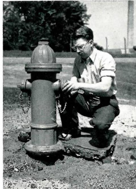
4 *After completing the inspection, replace nozzle caps correctly to avoid damage to threads. Simple, routine checks on hydrants will assure years of dependable, trouble-free service — at low cost.*
