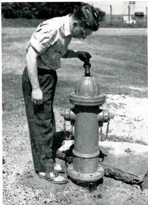
1 *Periodic examination and maintenance of hydrants should include a check of the oil reservoir. Operating nut of Mueller-Columbian hydrants can be removed for this purpose without shutting off water.*
