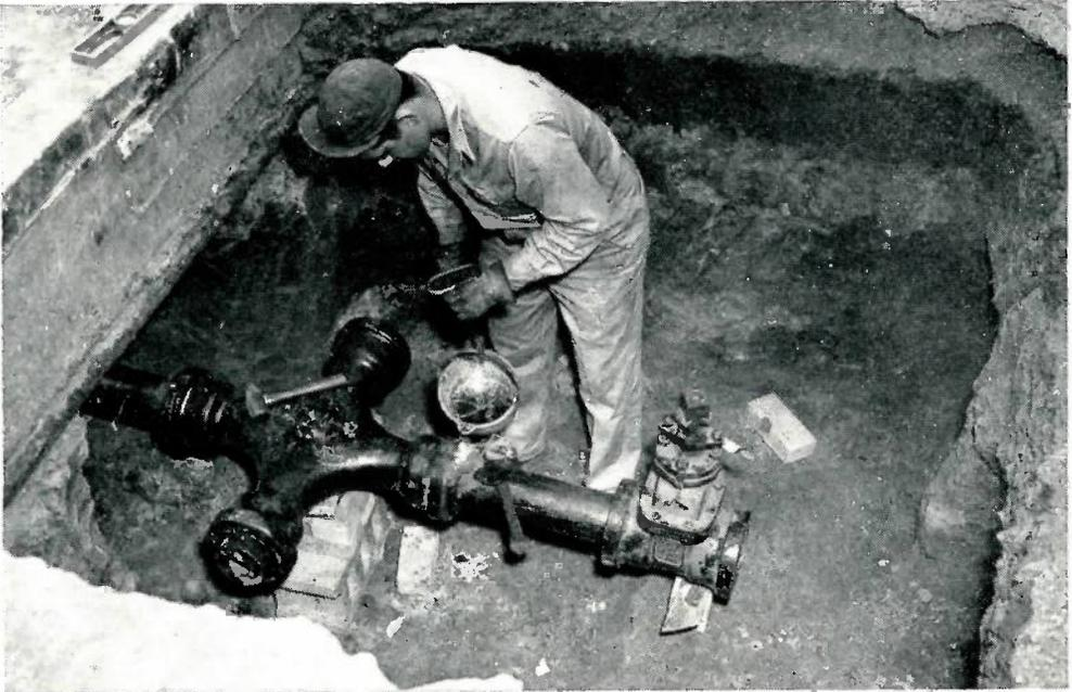
*R. W. Edwards, a plumber with George S. Walker, Inc., is shown leading a nipple into the bell end of the cross. A 4-inch Mueller gate valve is shown in the foreground of the photo.*
