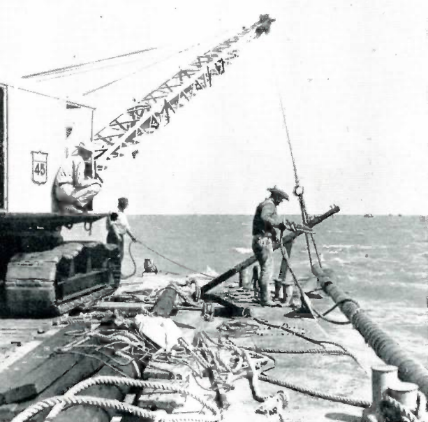
A war surplus LCT, carrying a tractor boom, was used as a working platform to join the end of the section already laid to the latest seaward addition.
