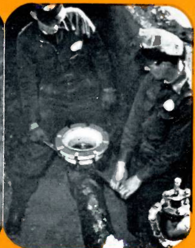
3. The valve adapter is securely bolted down on welded fitting.
