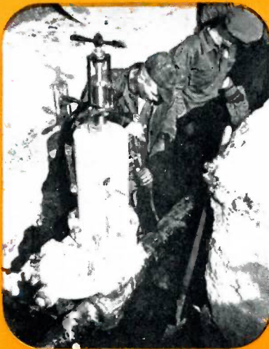
7. Stopper is pushed down in position shutting off the gas flow.
