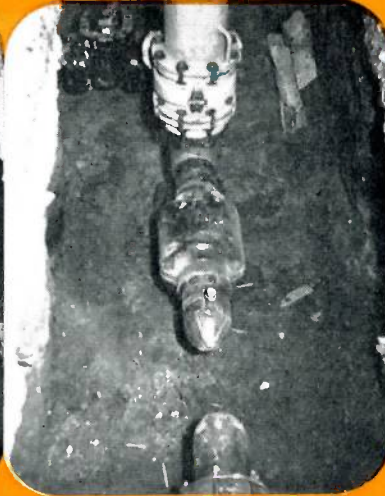
11. Completed job showing clamp welded in place, vent capped.
