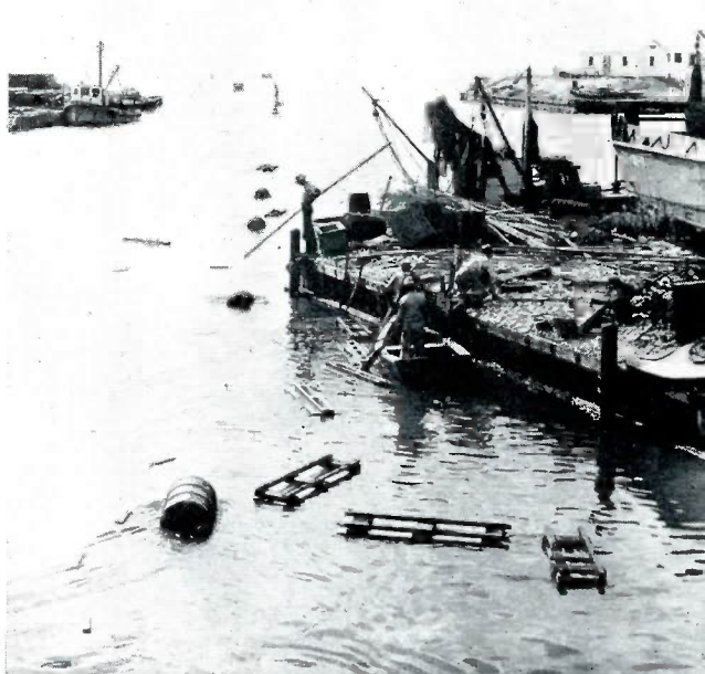
These floating oil drums support nearly a mile of pipe, submerged during towing. Tug, top center, can be seen towing a 5,000-foot section of the pipe line.
