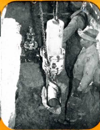
8. Rubber stopper is holding the pressure and the main is cut.
