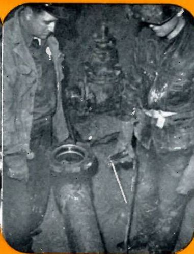
2. The fitting is now permanently welded in position on the line.
