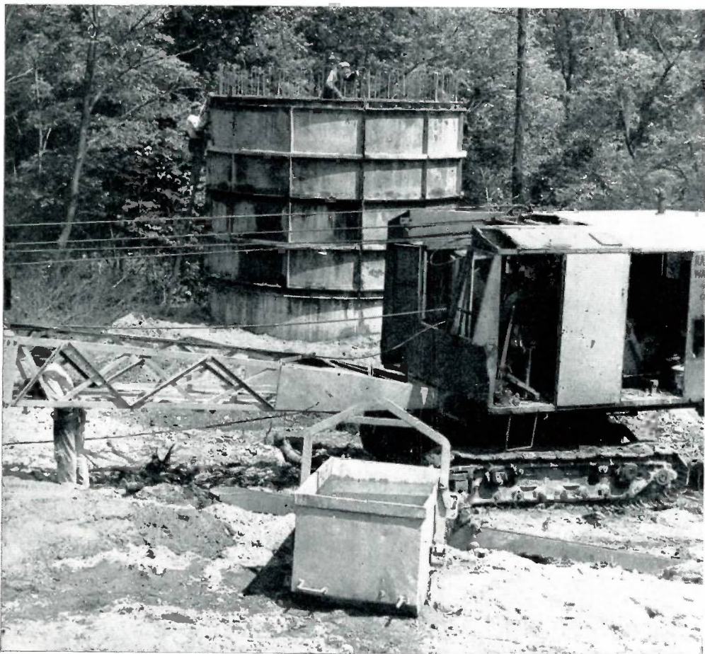
One of the three caissons built for the Canton system. Two serve as collector wells, feeding surface water to the underground reservoirs; the third is equipped with pumps for withdrawing the water. The system was built for a fraction of the cost of a surface dam.
