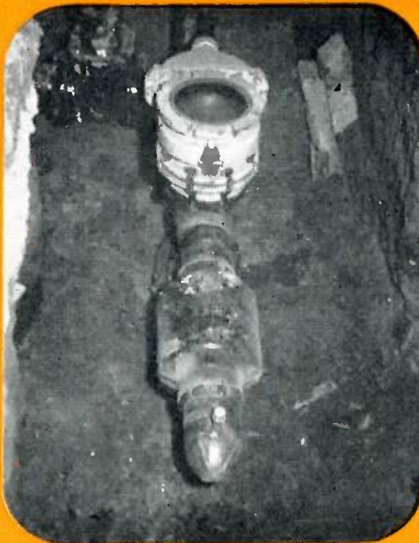
13. Stopping machine is removed; gate valve is holding pressure.
