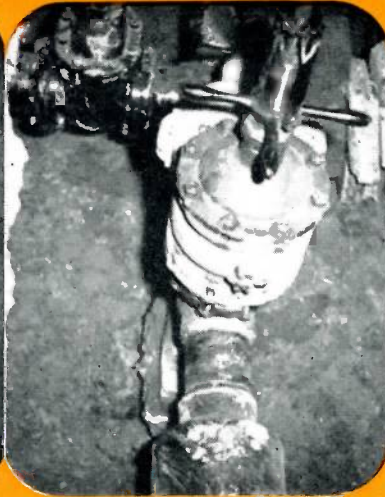
14. Completion plug is inserted by inserting and extracting machine.
