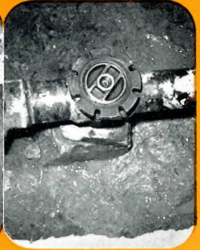
15. Threaded plug installed; completion cap is then bolted to fitting.
