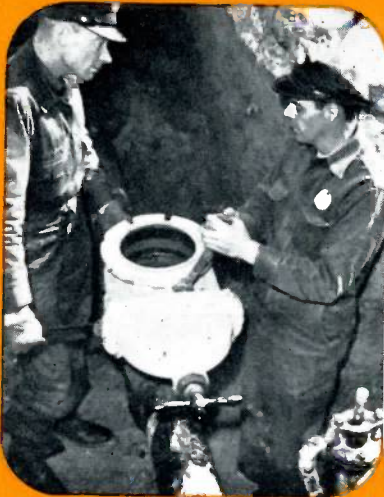
4. Gate valve is attached to the adapter ready for drilling machine.
