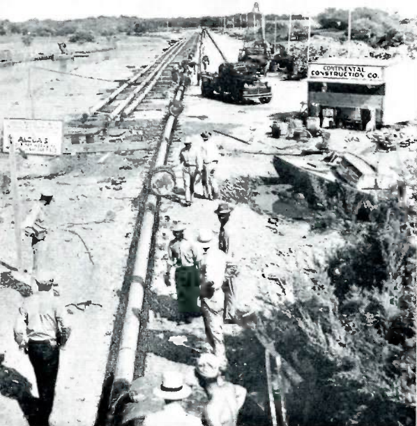
Along this 1,200-foot runway, 40-foot sections of pipe were welded into 1,000-foot sections, five of which were then welded together for towing into the bay.
