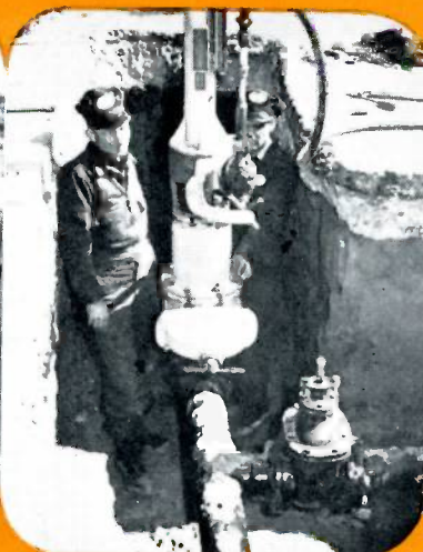
5. Cut is made into the line under pressure using a C-1 machine.
