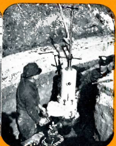
6. With gate valve closed, stopping machine is bolted to adapter.
