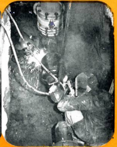
9. Installing clamp over coupling; bull plug is vented for safety.
