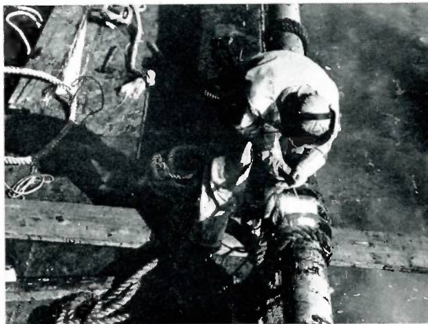
A Continental Construction Company welder on the LCT joins two 5,000-foot sections of the line at sea.
