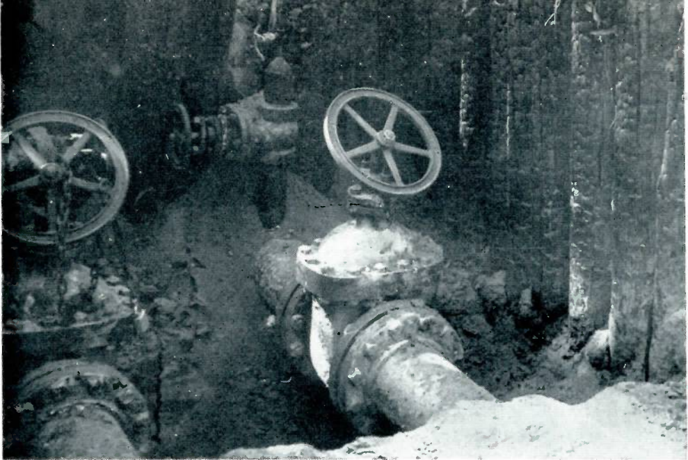
The damaged valves and wooden enclosure as they appeared after the fire.
