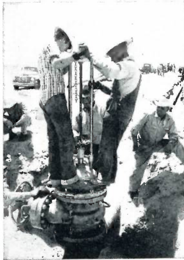
Expanding steel wedge stopper in H-17257 Line Stopper Fitting, making a complete stop-off.
