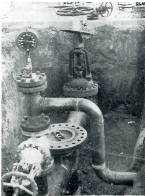
The valve is installed. Completion in place in line stopper fitting ready for completion cap. Note 1,000-pound pressure gage attached to by-pass connection.
