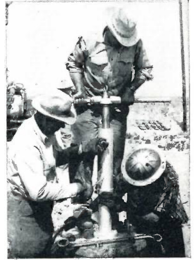
Inserting pressure equalizing "O" ring completion plug into Line Stopper Fitting, using H-17445 balanced pressure Completion Machine.
