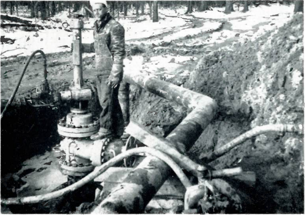
A Mueller C-1 drilling machine is drilling a ten-inch line stopper fitting through the special 14-inch gate valve. The eight-inch rigid by-pass line seen in the foreground was constructed to carry the load during the stopping operation.
