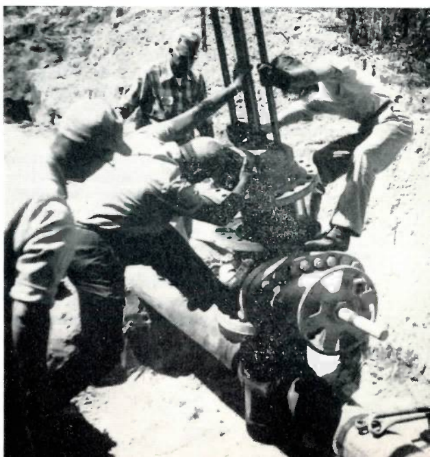
The workmen lower the No. 4 stopping machine in place on the valve.
