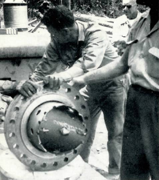
A C-1 drilling machine is removed with complete section of pipe retained in shell cutter.
