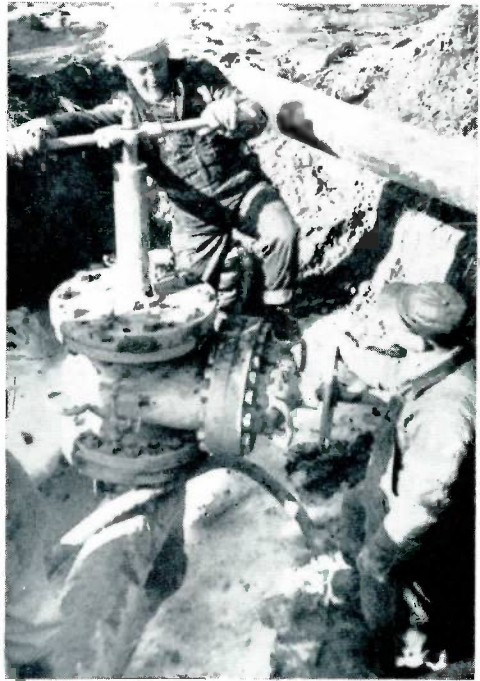
Inserting pressure equalizing completion plug using balanced pressure completion machine.
