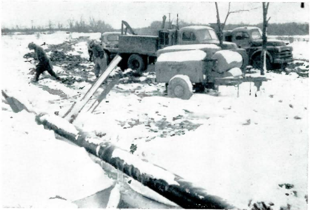
A general view of the site of operations. Note the general working conditions.
