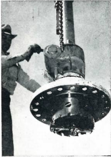
"C-1" Drilling Machine, with adaptor, removed from steel gate valve, showing section of pipe retained inside of shell cutter.
