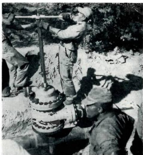
The steel wedge stopper is expanded off the line.
