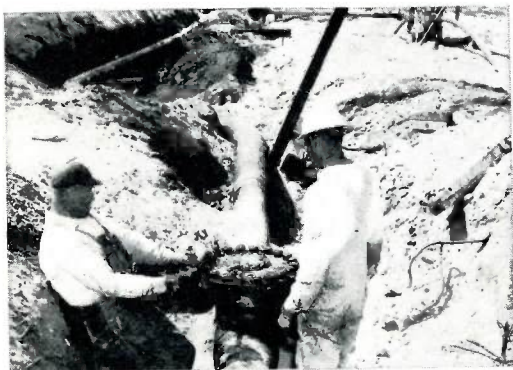
Completion Plug has been inserted into the Line Stopper Fitting and Completion Cap installed.
