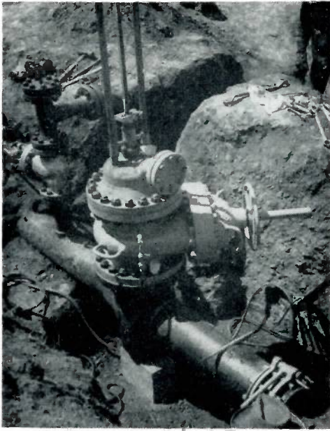
The old line is cut and ready for new valve.
