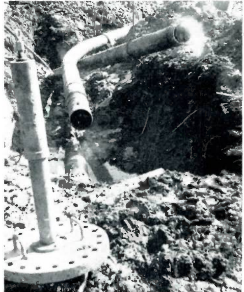
The old ten-inch line (upper right) has been cut and is being removed prior to lowering new line in place. Note vapor rising from cut section. Machine in foreground is the balanced pressure completion machine, part of Mueller No. 4 line stopper equipment.
