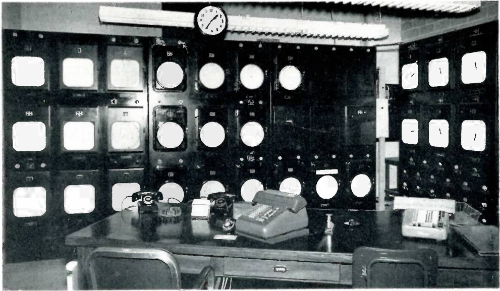
The company's modern, completely automatic central control system is pictured above. Shown at right is the newly-installed Bristol Telemetering Panel which shows at a glance the exact flow and pressure of gas along the Valley Gas distribution network. This automatic panel control system enables centrally-located dispatchers to determine and regulate gas supply according to demand throughout the system 24 hours a day.
