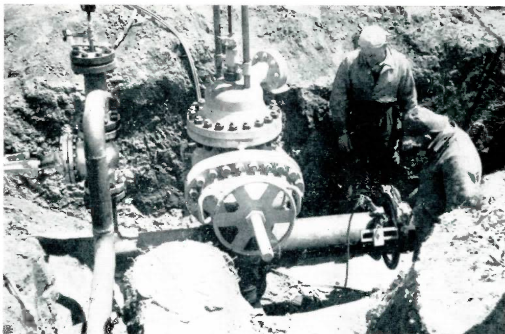
The steel wedge stopper is in place and expanded making tight shutoff. Pipe cutter cuts the pipe. The by-pass is shown at left center.
