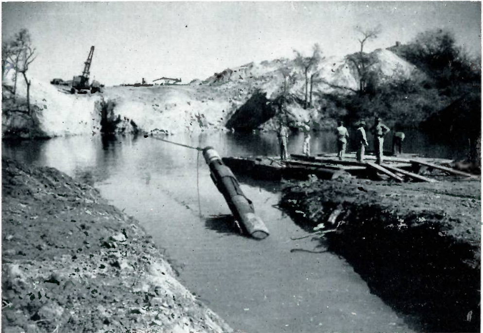
One of the lines being pulled across the Guadalupe River near New Braunfels, Texas. The dual underwater crossing is part of a construction project of United Gas Pipe Line Company to increase deliveries of natural gas to customers in the New Braunfels-Austin area.
