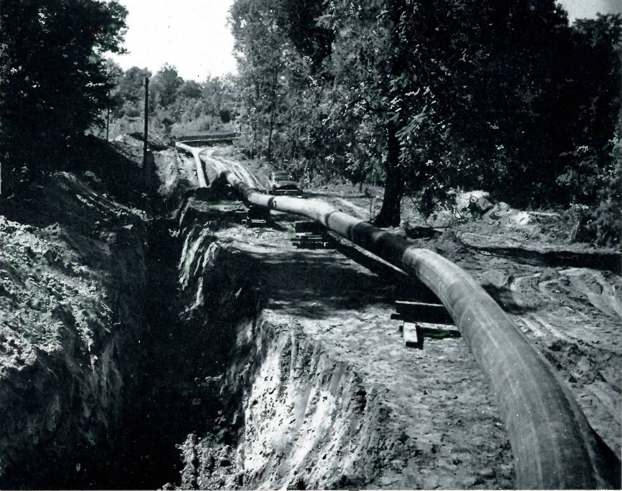
Here's Arkansas Louisiana Gas Company's 20-inch natural gas line ST-1 under construction. It extends from Carthage, Texas, to Waskom, Texas.
