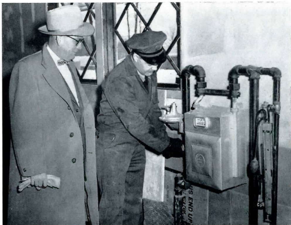
Otto Shook of the Ohio Fuel Gas Co. service department completes procedures which begin the flow of natural gas into the first house in the United States to undergo tests to determine whether an average size American home can be heated and cooled for $120. Walter Weirich, service manager, looks on.
