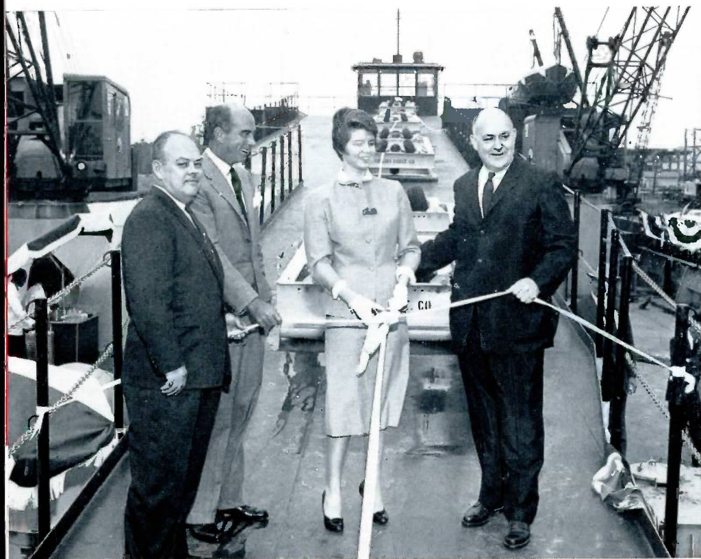
Jo Ann Liese, daughter of Commonwealth Oil Company president G. Burton Liese, is shown cutting the ribbon, officially commissioning the offshore industry's first specially-built pipe-laying barge, the "Magic."
