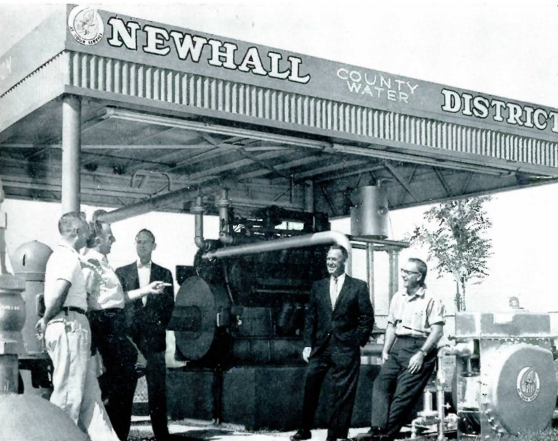
The performance of this natural gas-fired engine drew high praise from area water district officials. Discussing the merits of the engine are (left to right): District Manager O. L. Martin, Board of Directors President E. W. Nichols, Roger Morey, C. A. Akins, and Dale Taylor. All except Mr. Akins, who is with the Southern California Gas Company, are with the Newhall Water District in Los Angeles County.
